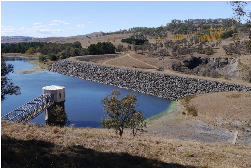
Figure 13: View of Malpas Dam spillway and intake tower
