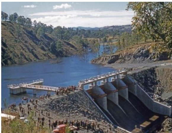
Oaky River Dam Opening in 1956 (pre-failure), looking upstream.
