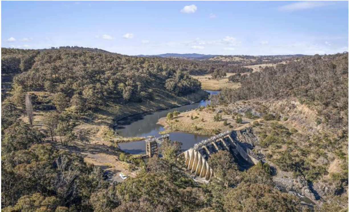
Figure 12: Aerial view of damaged Oaky River Dam wall
