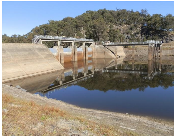
Oaky River Dam Pre-failure.
