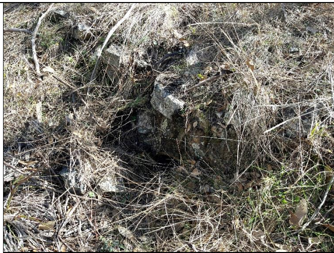
Character of rock culvert recorded.
