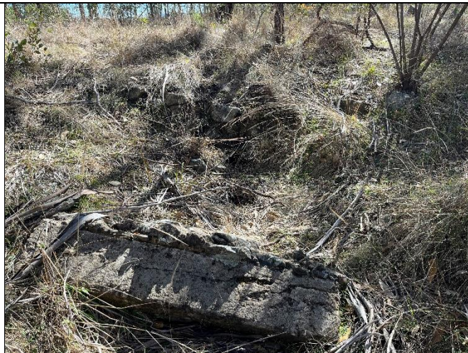
Character of rock culvert recorded.
