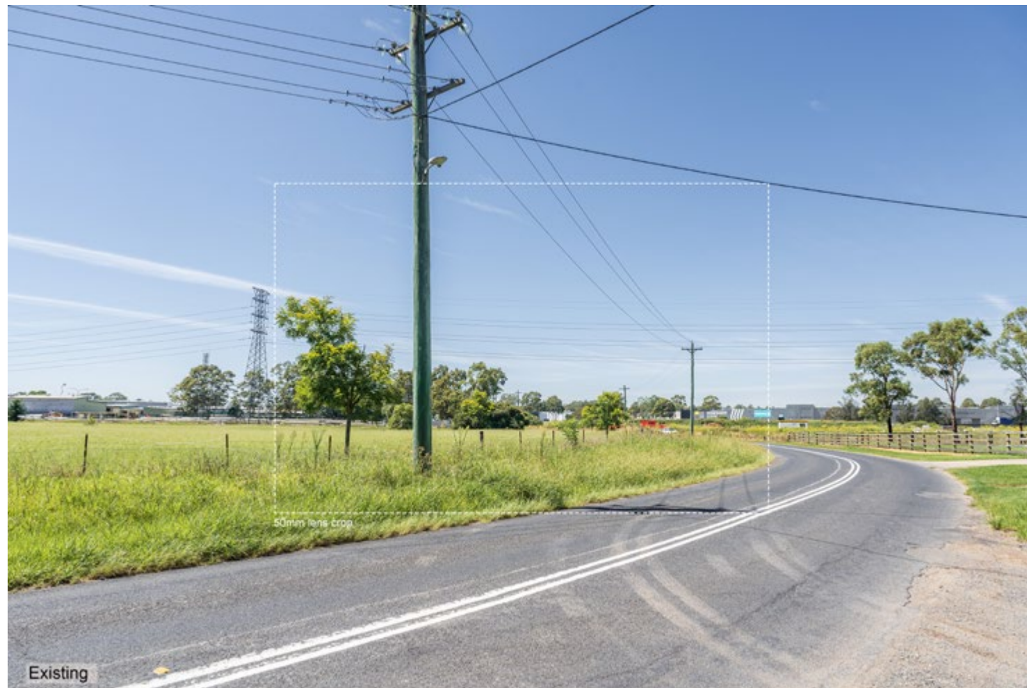
Existing View: Blaikie Road (West)
