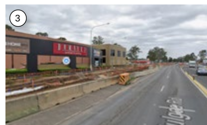
View from Mulgoa Road looking North-East
