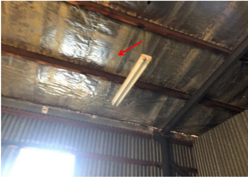
Photograph 65: HAZCHEM shed, internal , roof, insulation material, SMF identified visually.
