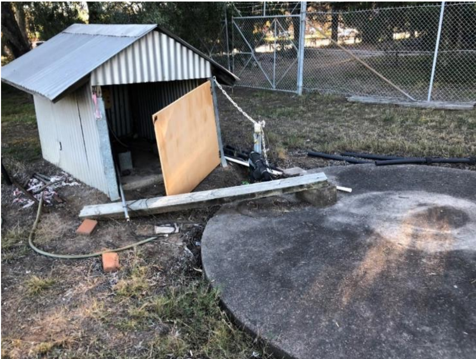
Photograph 20: Concrete water tank (in ground).
