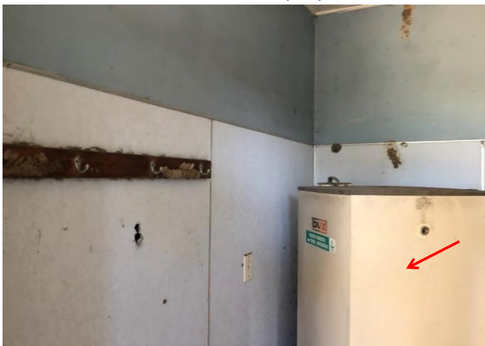
Photograph 59: Rear Office, internal , wet room, walls, lower half (marbled finish), fibre cement sheet, asbestos detected by analysis.
