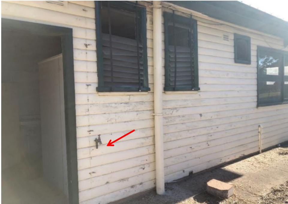
Photograph 51: Rear Office, external, walls, beige paint, lead paint (>0.1% lead w/w).
