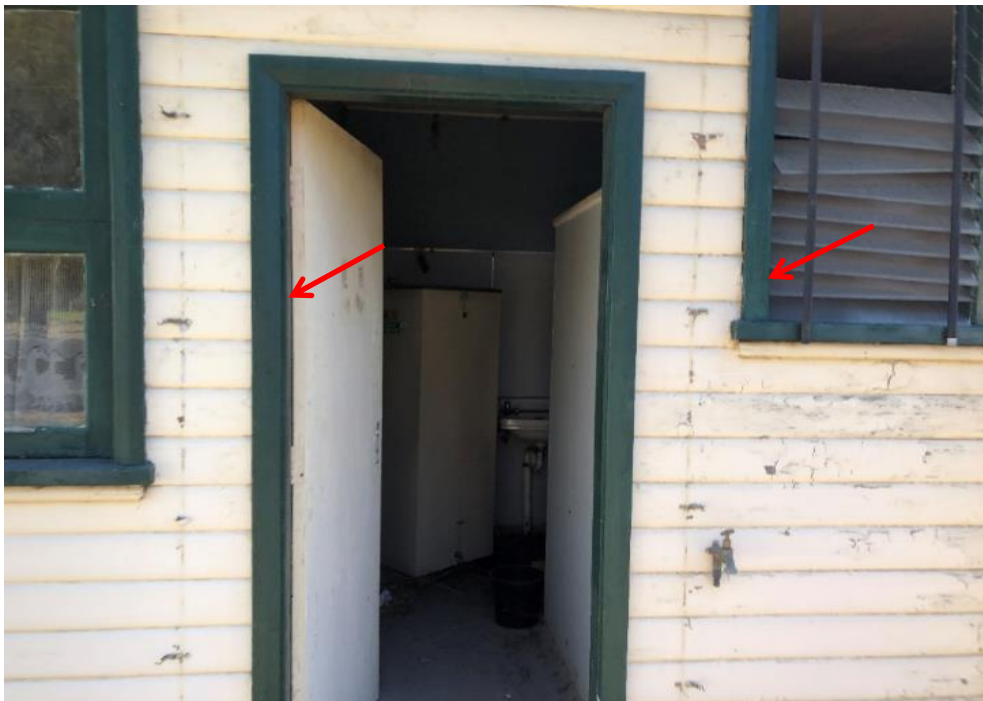
Photograph 51: Rear Office, external, walls, beige paint, lead paint (>0.1% lead w/w).
