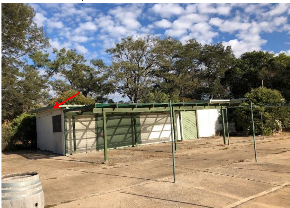
Photograph 38: Front Office, external, eaves, fibre cement sheet, no asbestos detected by analysis.
