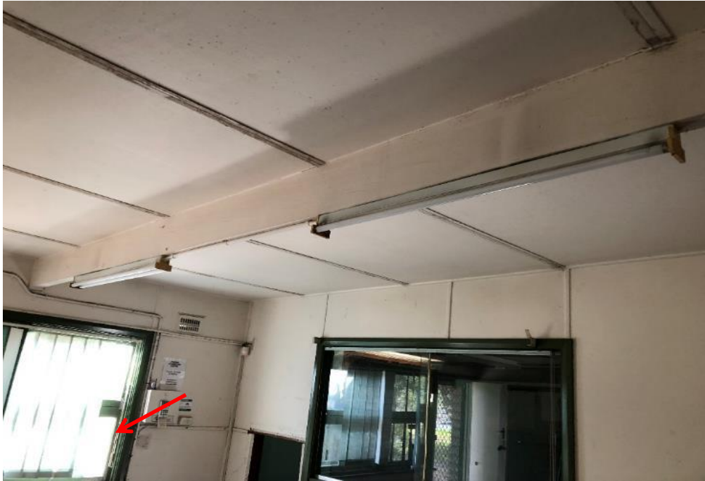
Photograph 45: Front Office, internal , windows and architraves, green paint, non-lead paint (≤0.1% lead w/w).
