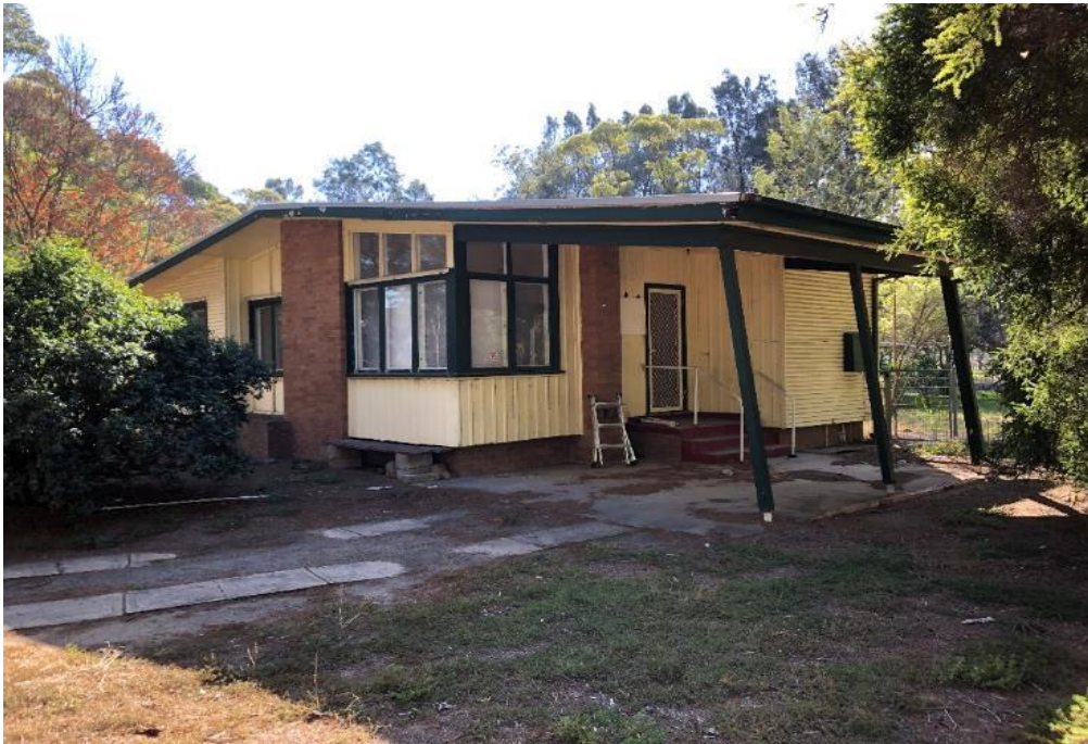
Photograph 1: Building 1 - Timber framed residential dwelling with timber floors and skillion roof
