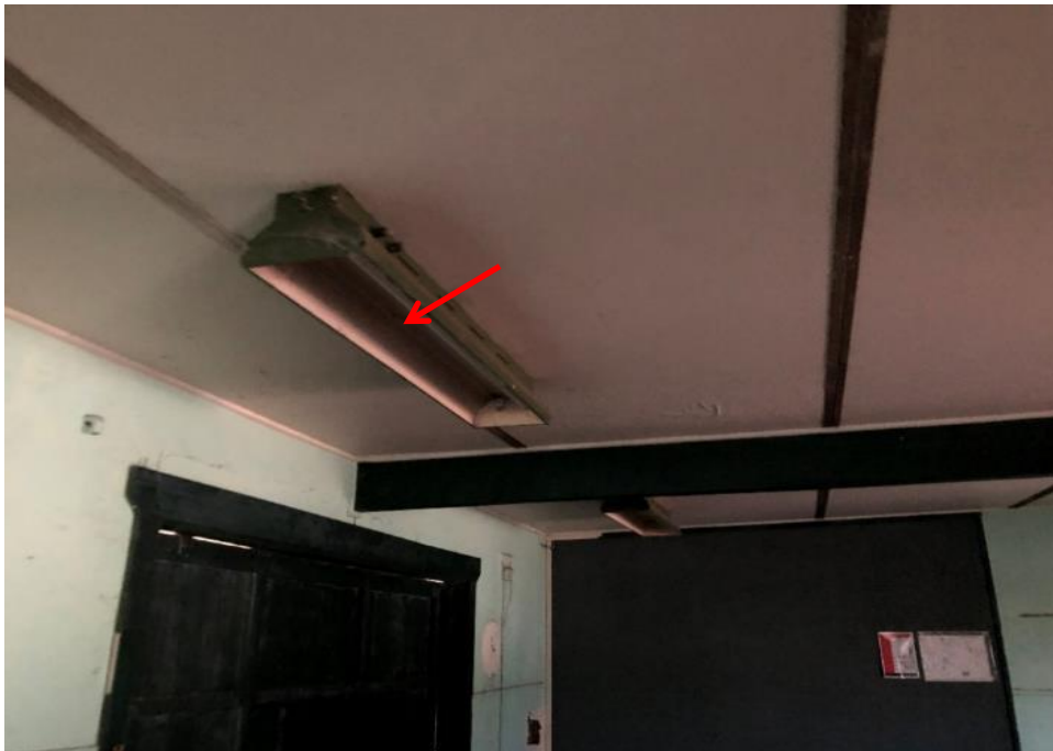
Photograph 43: Front Office, internal , fluorescent light fittings, capacitors, insulating oil, PCB (assumed).
