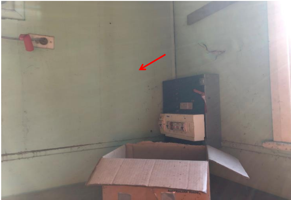
Photograph 57: Rear Office, internal , walls, fibre cement sheet, asbestos detected by analysis.
