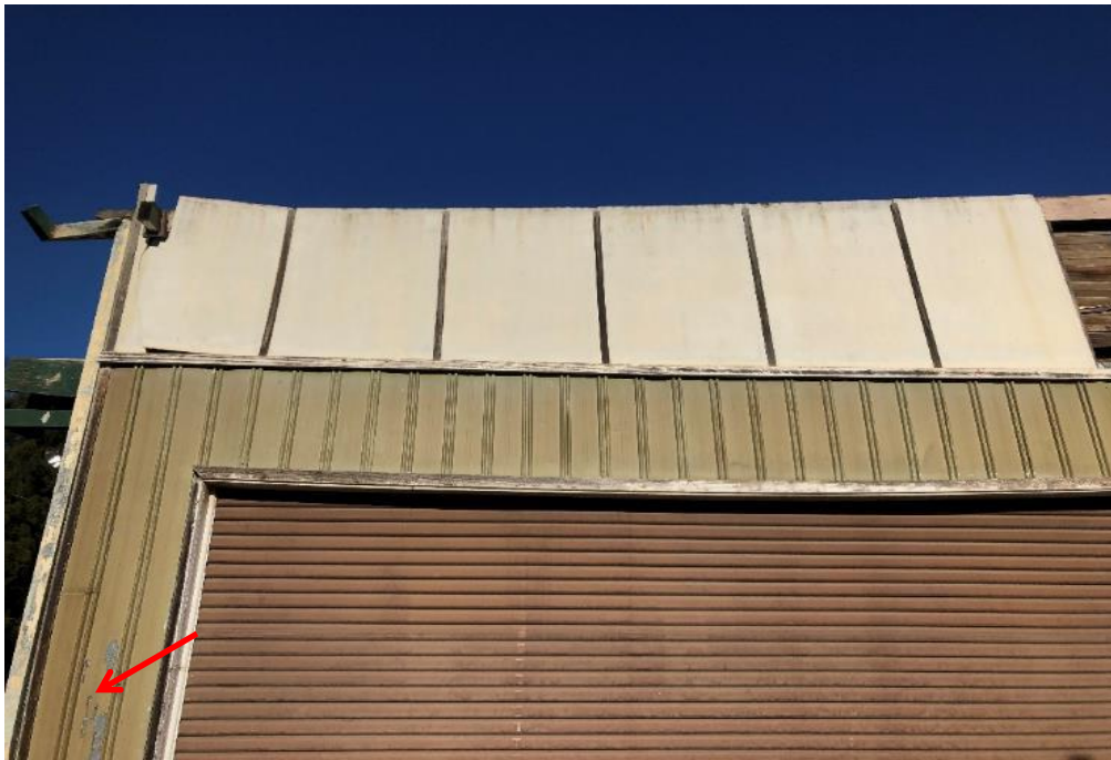
Photograph 23: Potting shed, external , corrugated sheet metal, green paint, lead paint (>0.1% lead w/w).
