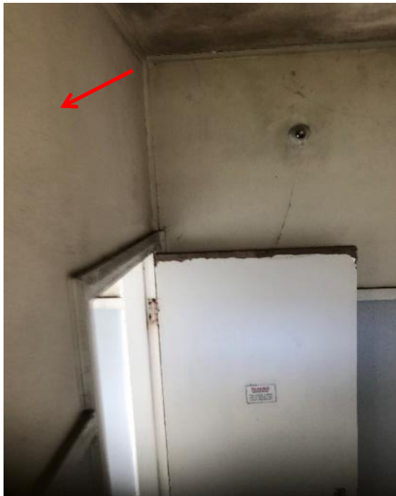
Photograph 39: Front Office, external, walls, cream paint, non-lead paint ( \leq 0.1\% lead w/w).
