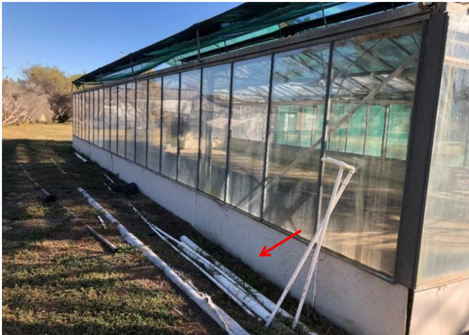
Photograph 67: Glasshouse, external , walls, fibre cement sheet, no asbestos detected by analysis.
