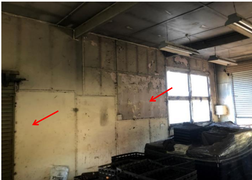
Photograph 33: Potting shed, internal , potting shelf, fibre cement sheet, no asbestos detected by analysis.
