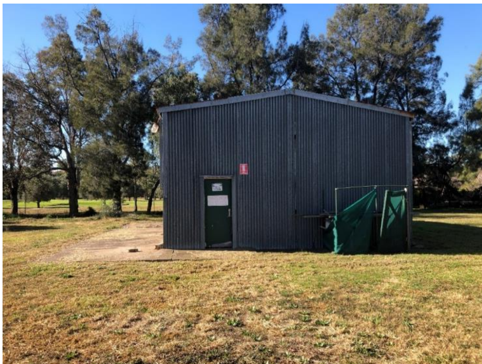
Photograph 62: Machinery and HAZM/CHEM shed.
