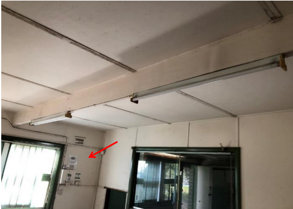
Photograph 41: Front Office, internal , wall cavities, insulation material, SMF (assumed).
