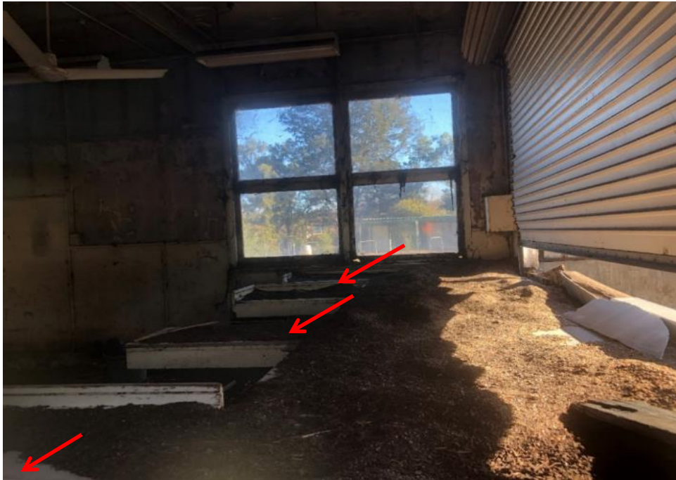
Photograph 33: Potting shed, internal , potting shelf, fibre cement sheet, no asbestos detected by analysis.
