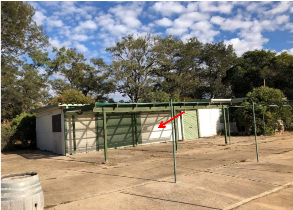
Photograph 39: Front Office, external, walls, cream paint, non-lead paint ( \leq 0.1\% lead w/w).
