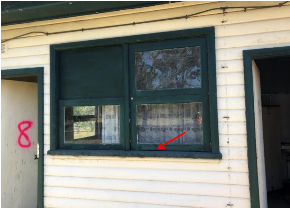
Photograph 53: Rear Office, external , windows, putty, no asbestos detected by analysis.
