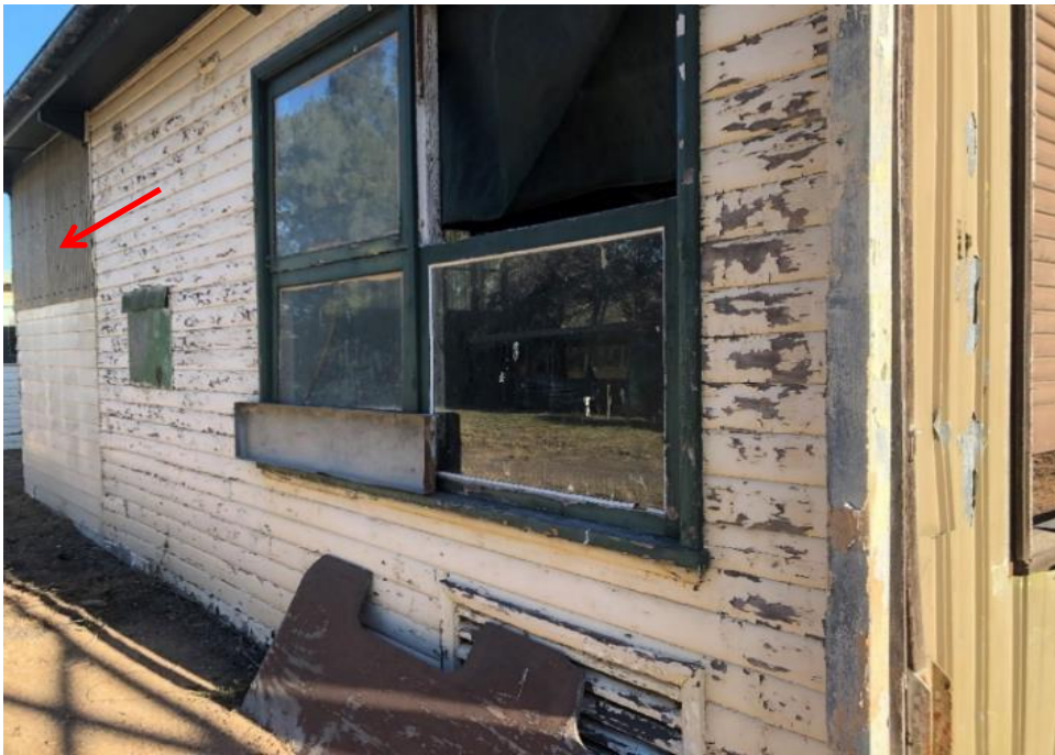
Photograph 31: Potting shed, external , walls, corrugated sheeting, SMF (assumed).
