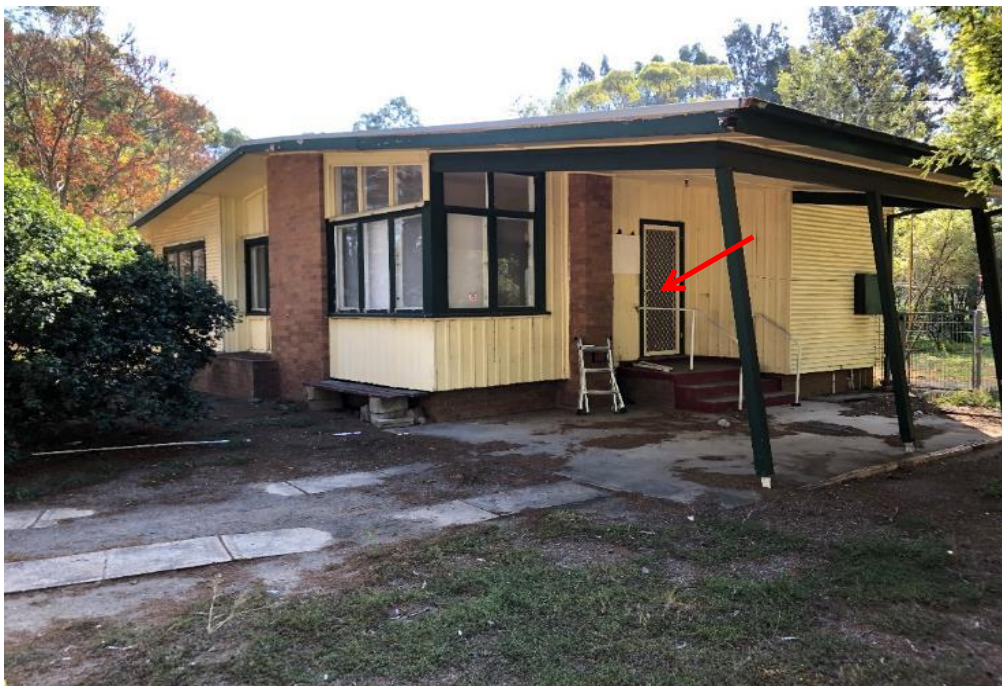
Photograph 14: Residential Dwelling, external , front door, cream paint, non-lead paint (≤0.1% lead w/w).
