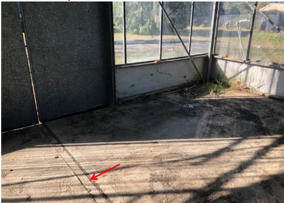
Photograph 67: Glasshouse, external , walls, fibre cement sheet, no asbestos detected by analysis.
