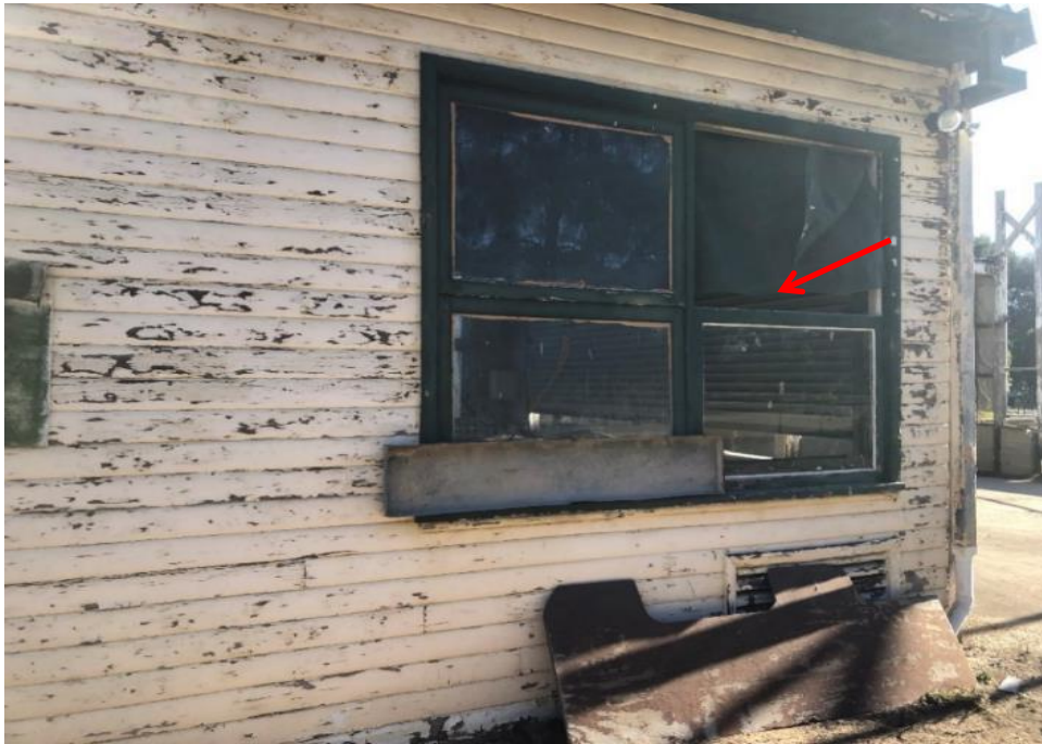
Photograph 27: Potting shed, external , windows, putty, non-lead paint ( \leq 0.1\% lead w/w).
