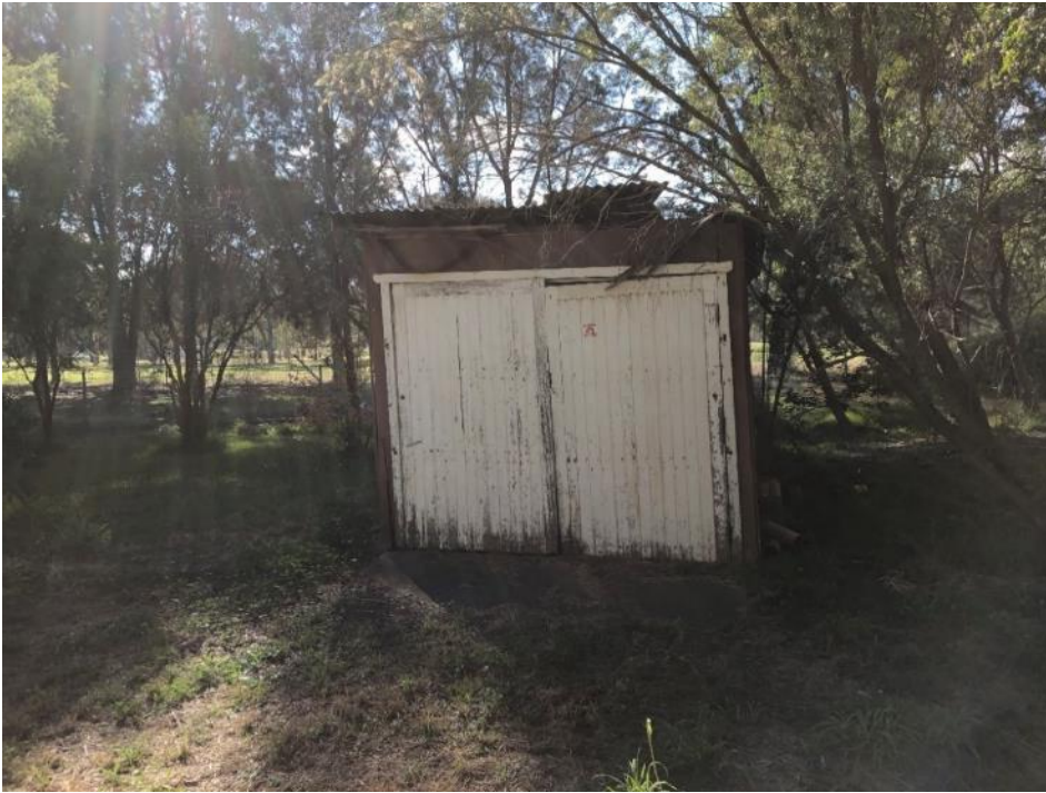
Photograph 17: Timber shed to rear of residential dwelling.
