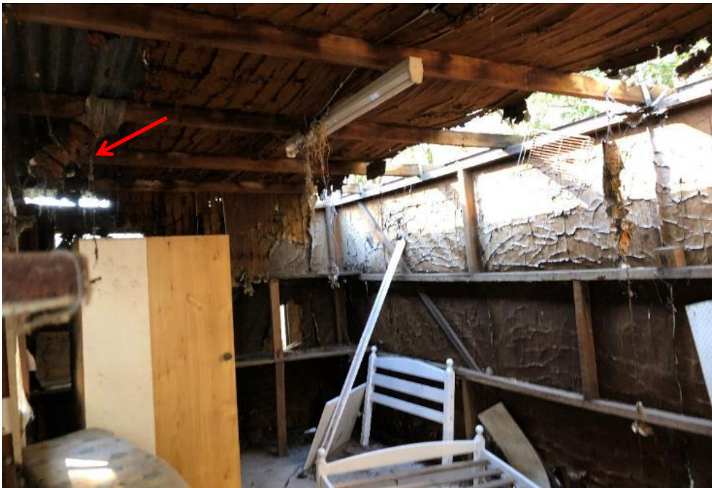
Photograph 18: Rear Shed, roof, insulation blanket, insulation, SMF (assumed).
