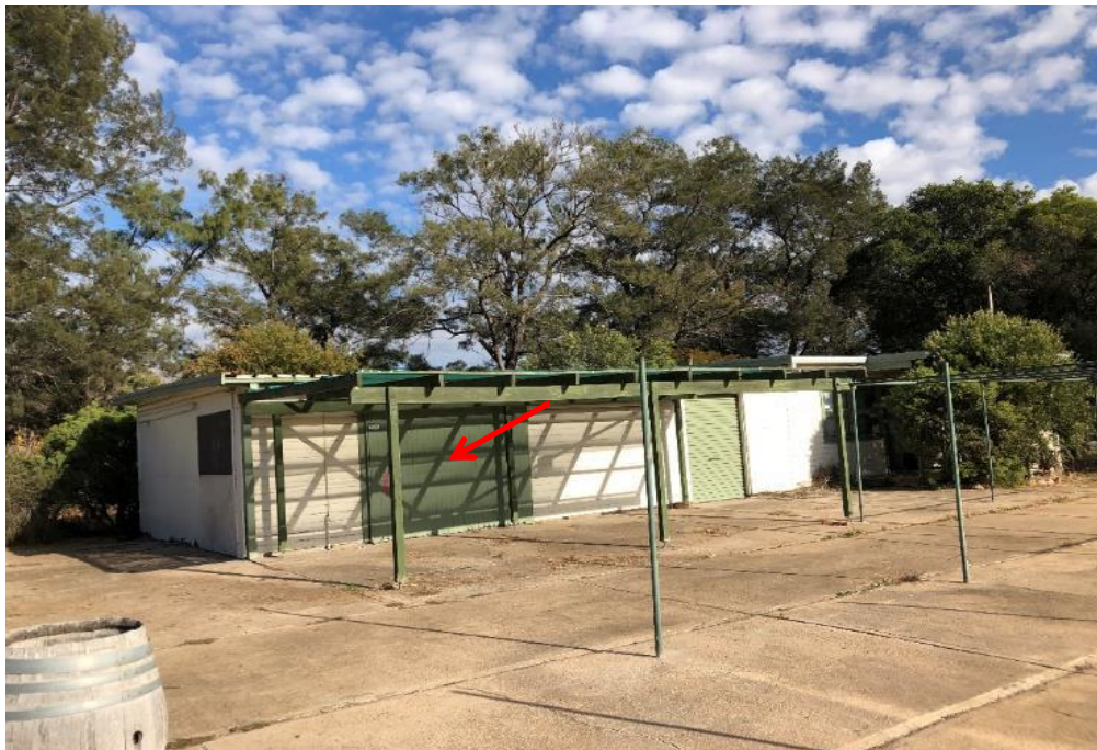
Photograph 37: Front Office, external, sliding door, pale green paint, non-lead paint ( \leq 0.1\% lead w/w).
