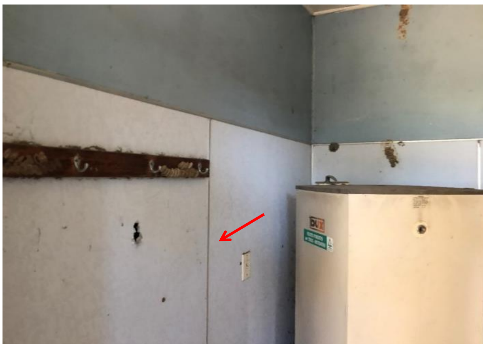
Photograph 59: Rear Office, internal , wet room, walls, lower half (marbled finish), fibre cement sheet, asbestos detected by analysis.
