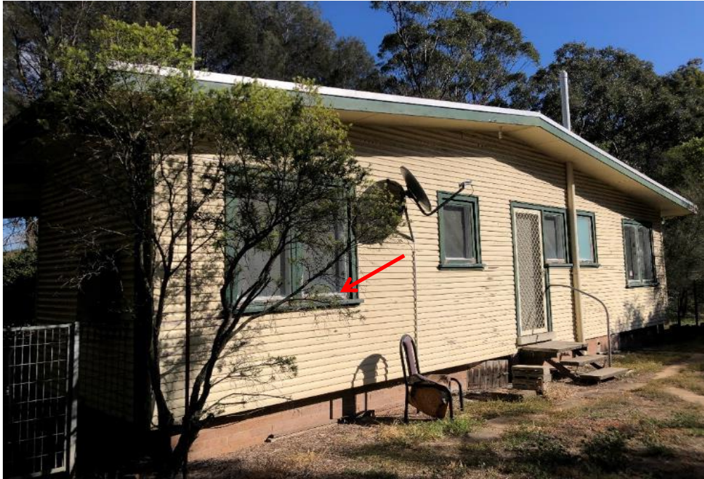
Photograph 9: Residential Dwelling, external , windows, putty, no asbestos detected by analysis.
