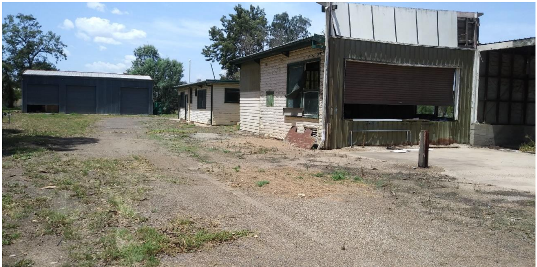
Figure 9 Structures on site
