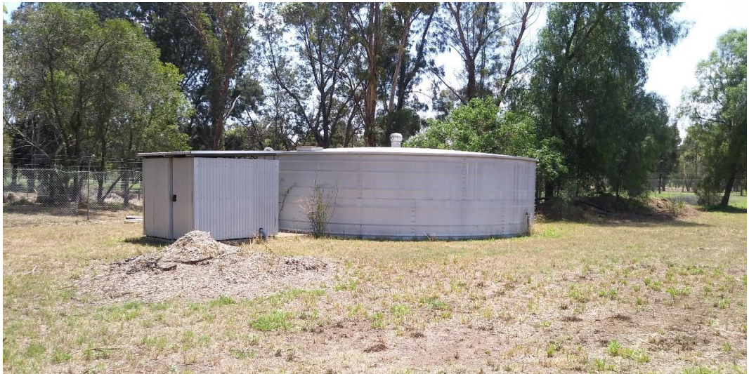
Figure 11 Structures on site
