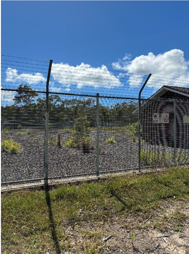
Figure 4: Former substation yard
