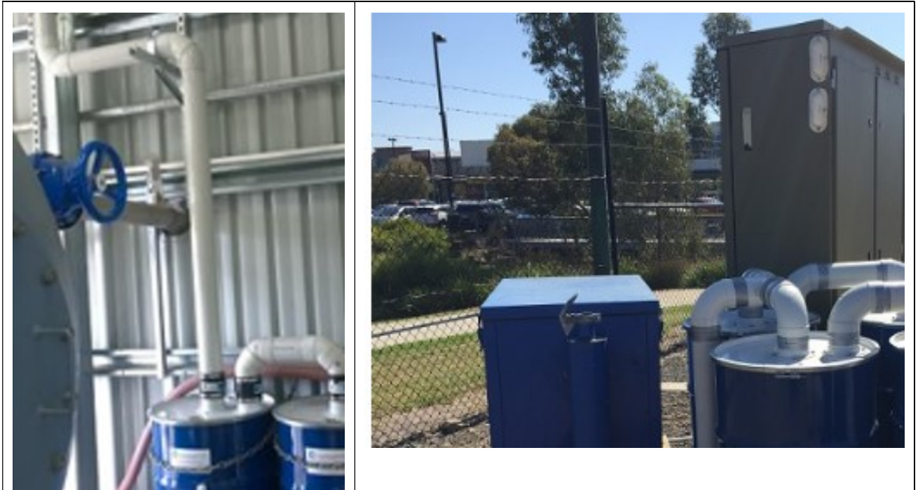
Figure 5.6 Granular Activated Carbon (GAC) Canisters for Air Filtration. Modular system allows all offensive gases to be scrubbed, and additional canisters installed if required.
