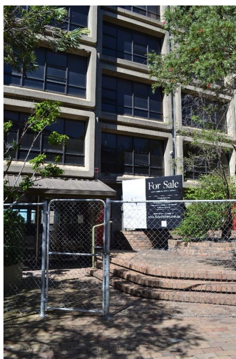
Figure 7 View of the existing entrance to the Sirius building from Cumberland Street Source: Architectus
