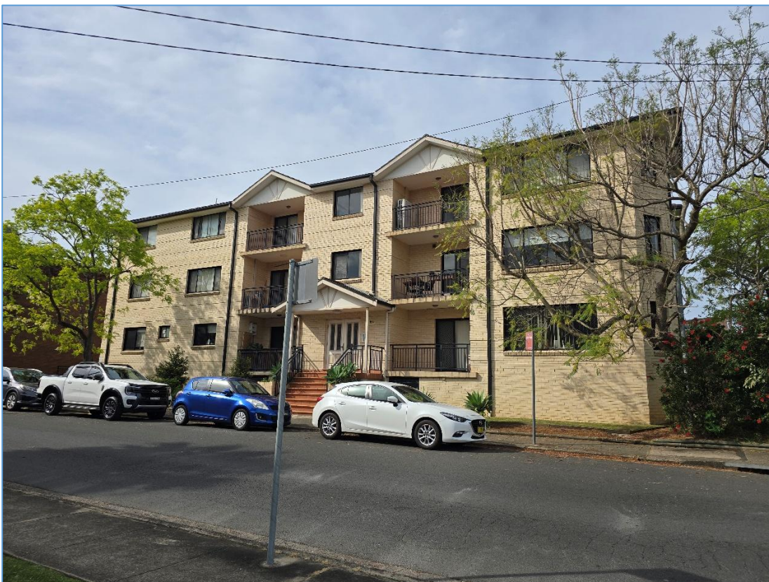
Figure 3 Residential flat building at 56 Pitt Street
