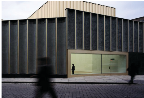
Podium expression with pre-cast concrete sheeting.
