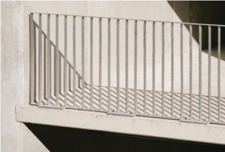
Steel balcony railings, to open up facade.
