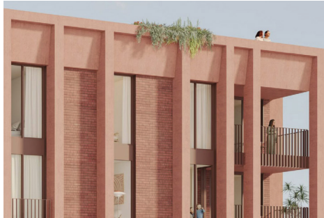
Podium expression with setback brick wall, and protruding concrete columns.
