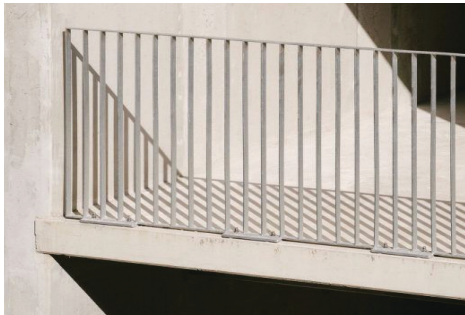
Steel balcony railings, to open up facade.
