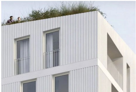
Metal fluted wall panelling on a facade.
