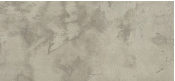
Finished Concrete Balcony Flooring
