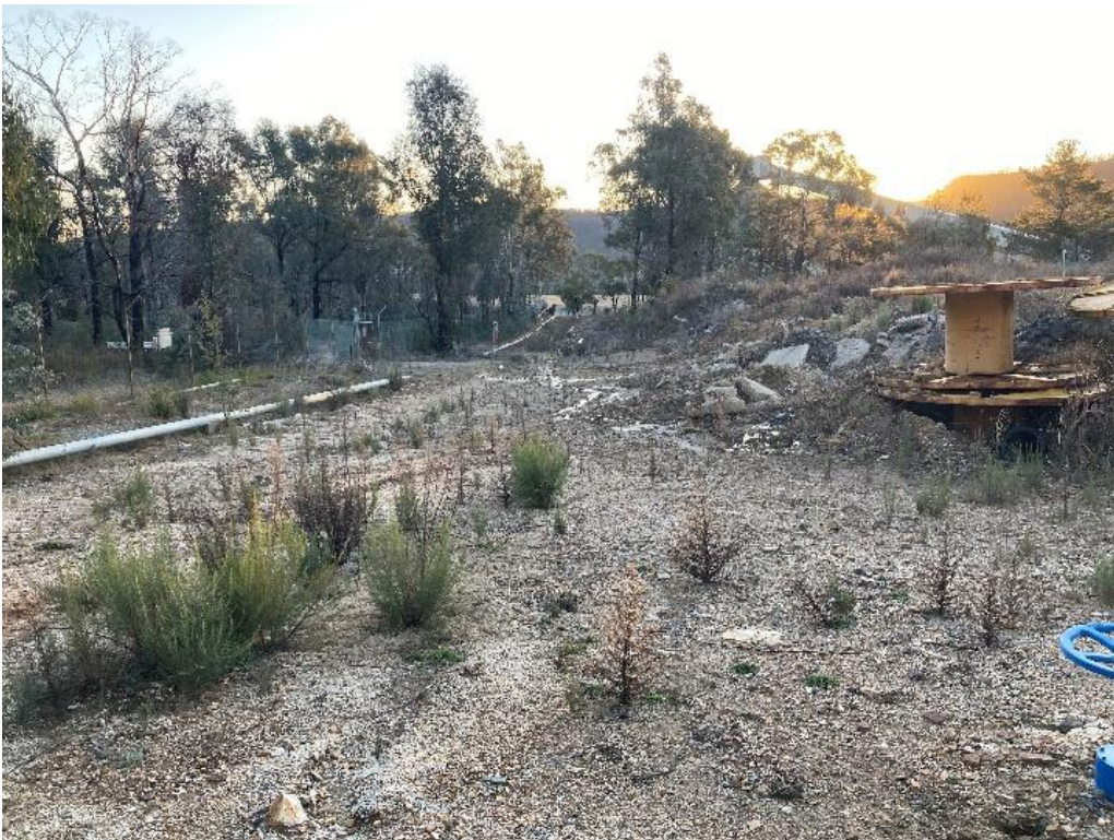
Photograph 4.1 Pipeline disturbance footprint
