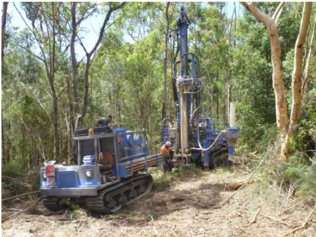
Photograph 9: Mantis 300 rig with air compressor during aircore drilling on DMAC01.
