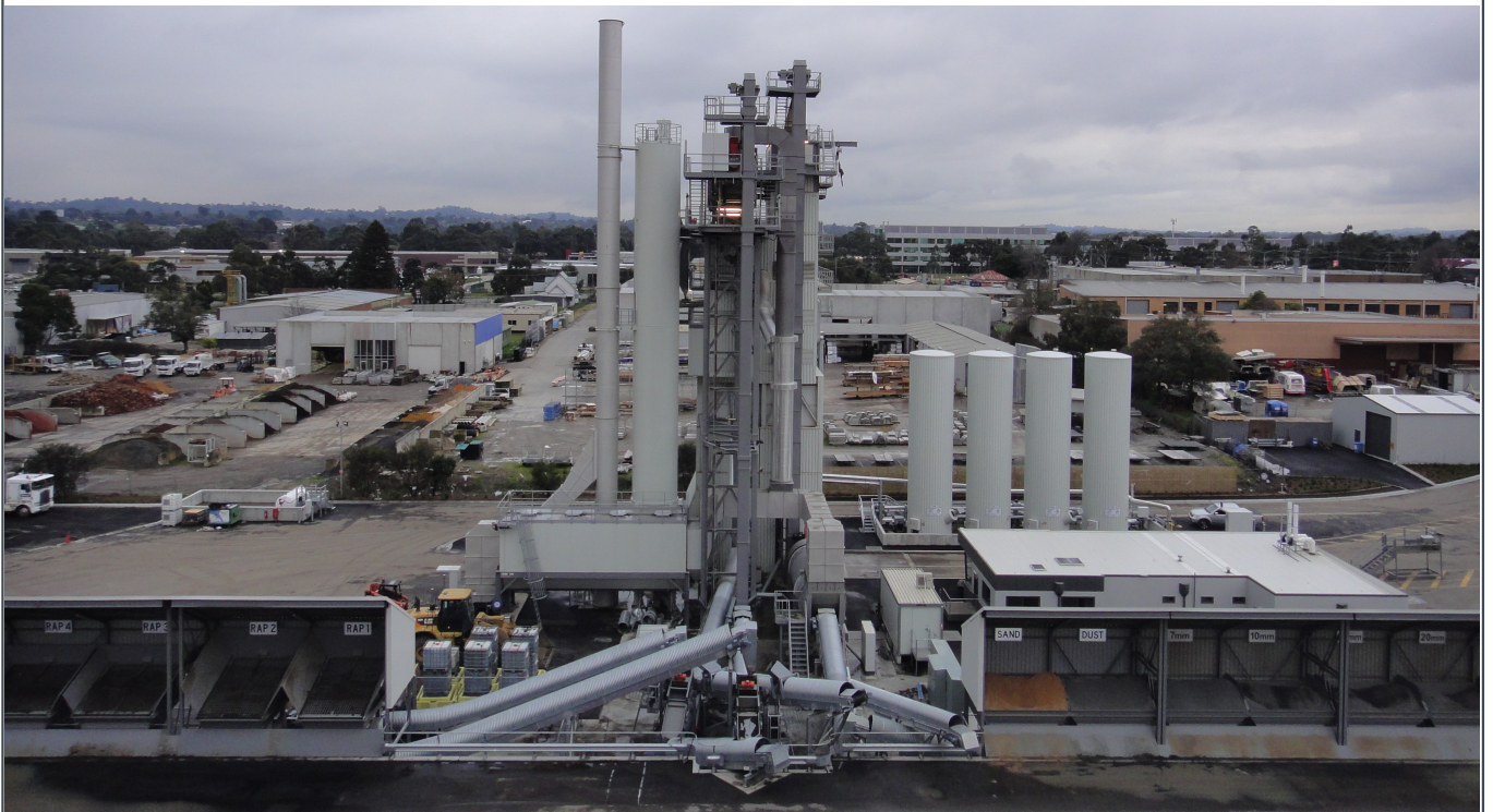
F2.3b: Photograph of similar asphalt plant
