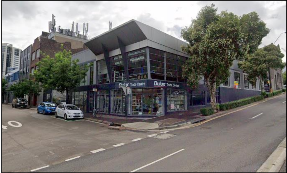
Figure 5 Development to the Immediate North Looking North East Source: Google
