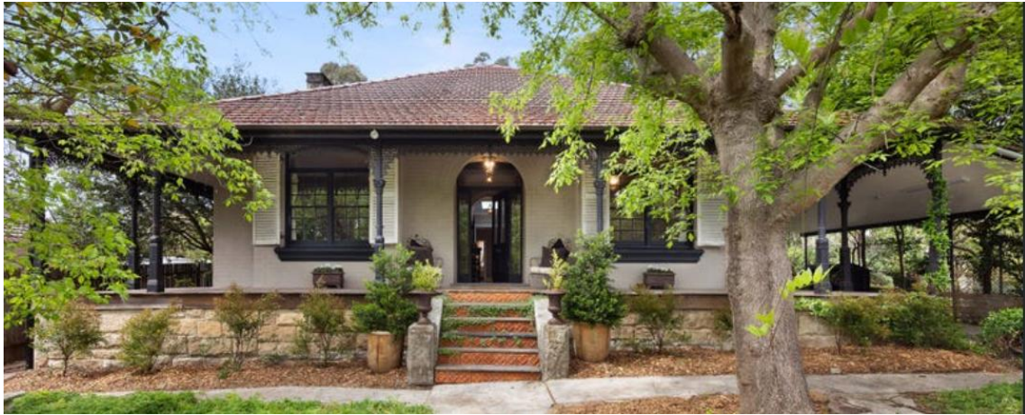
Figure 12: Front elevation of No. 19 McIntosh Street, Gordon
