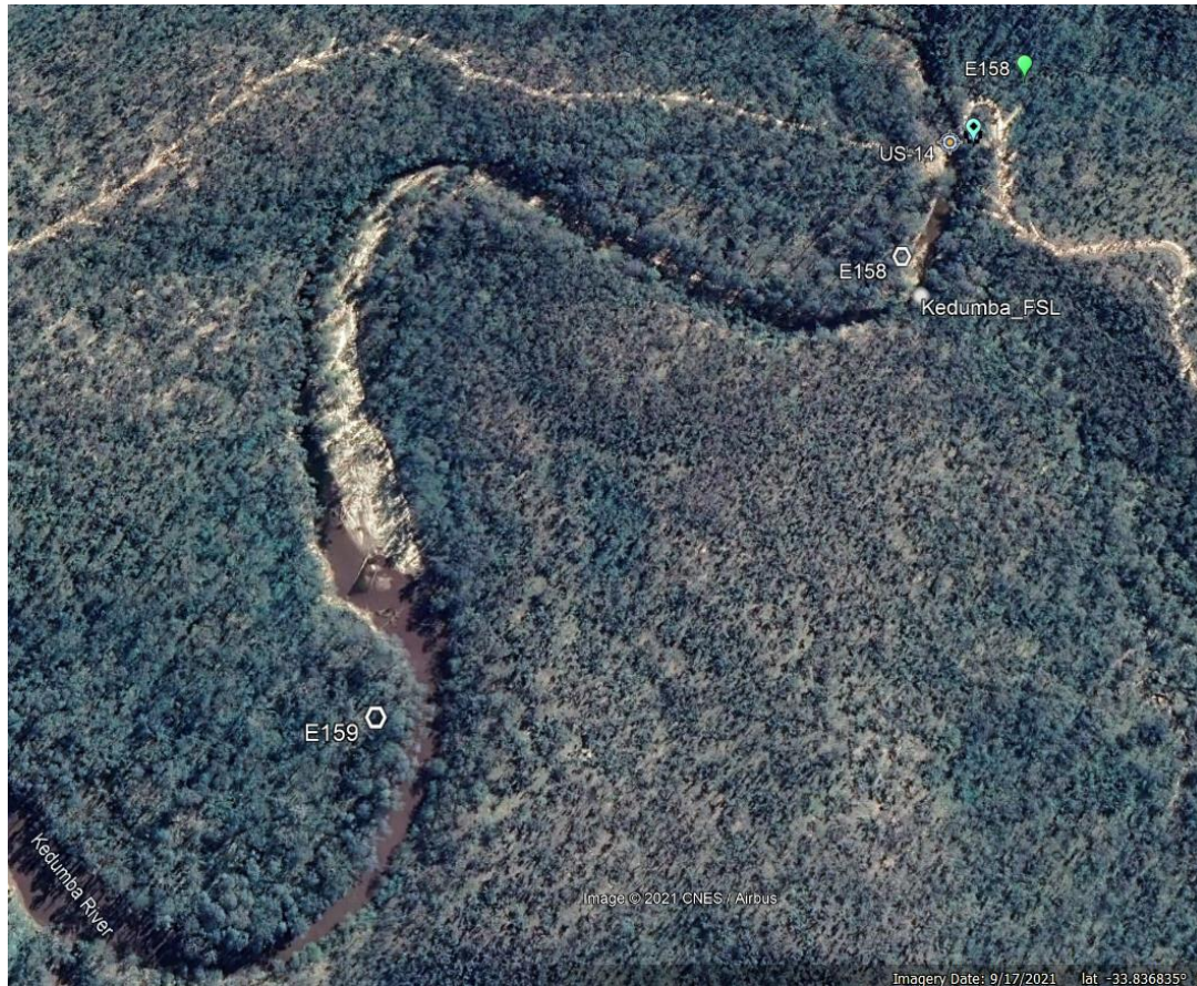
Figure 11. Effects of inundation in the lower Kedumba River.
