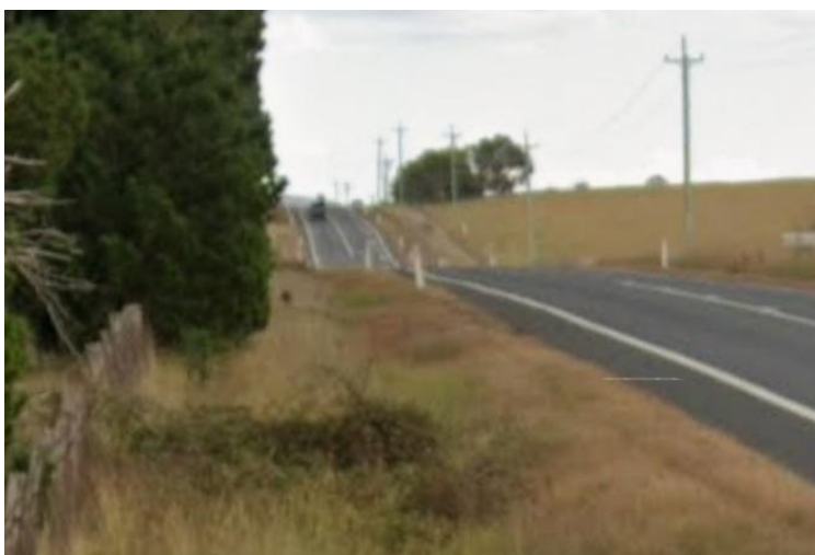
Figure 1: Crest on Braidwood Road, looking south from Painters Lane intersection. (Source: Google Maps)
