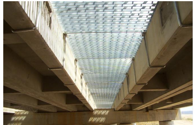
View under the bridge at Lakes Environs (Waterside Green) looking up at a grate incorporated into the structure
