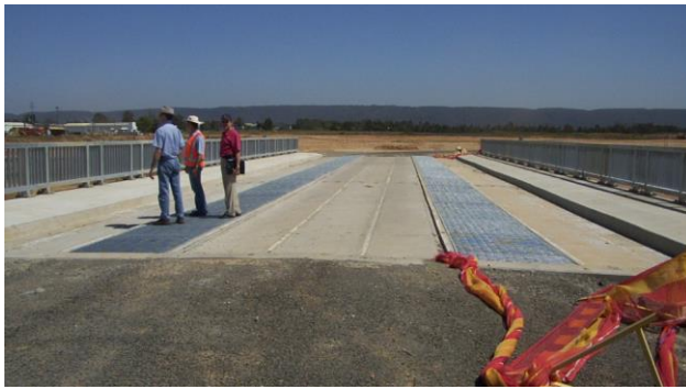
An example of a bridge at Lakes Environs (Waterside Green), Lakeview Drive Cranebrook with grates incorporated into the structure to assist in allowing light and moisture penetration for plant growth under the bridge
