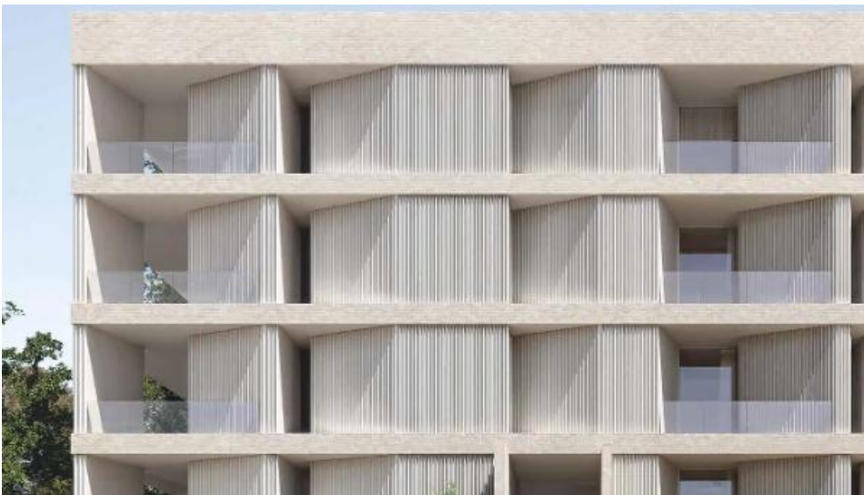
Figure 9 – Example of pleated metal cladding contained within a solid frame
