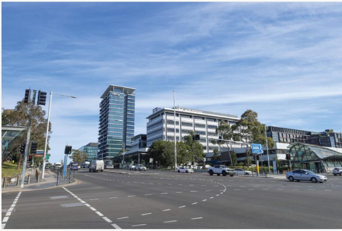
Existing site photo
