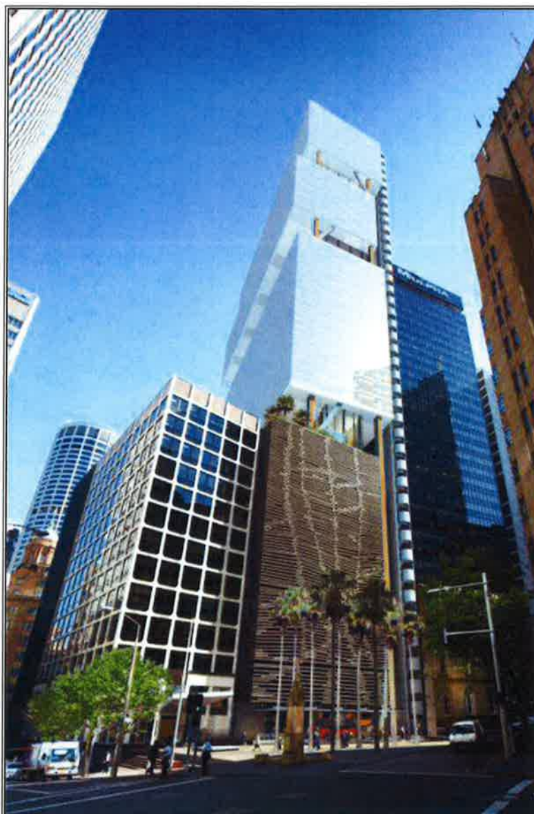
Figure 4: View west to the Bligh Street elevation of the substation and Integrated Commercial Tower (Source: Project Approval)
