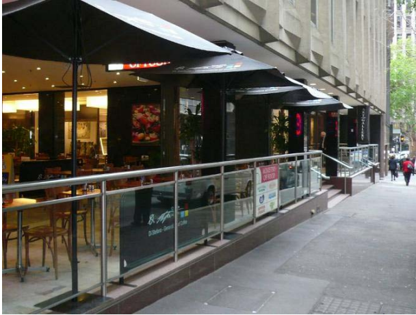
Relatively recently installed café on the Bligh Street frontage of the office building next to the early 1970s former Wentworth Hotel, almost opposite subject site.
