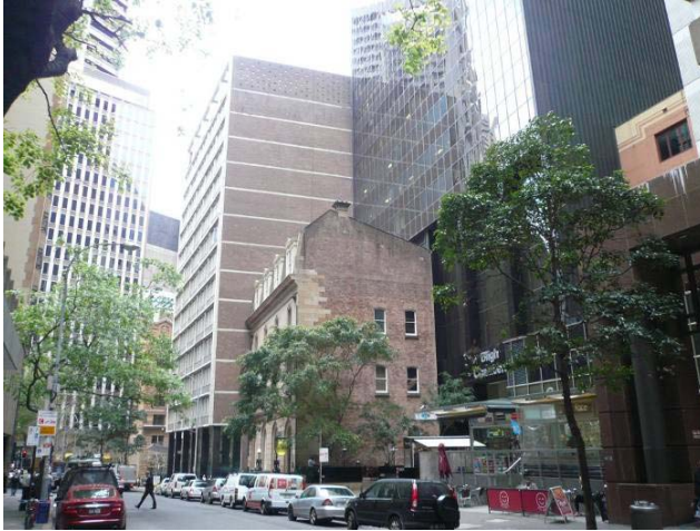
View down Bligh Street past the mini-plazas to the side elevation of the former NSW Club building. Kindersley House, on the subject site forms the medium rise backdrop.
