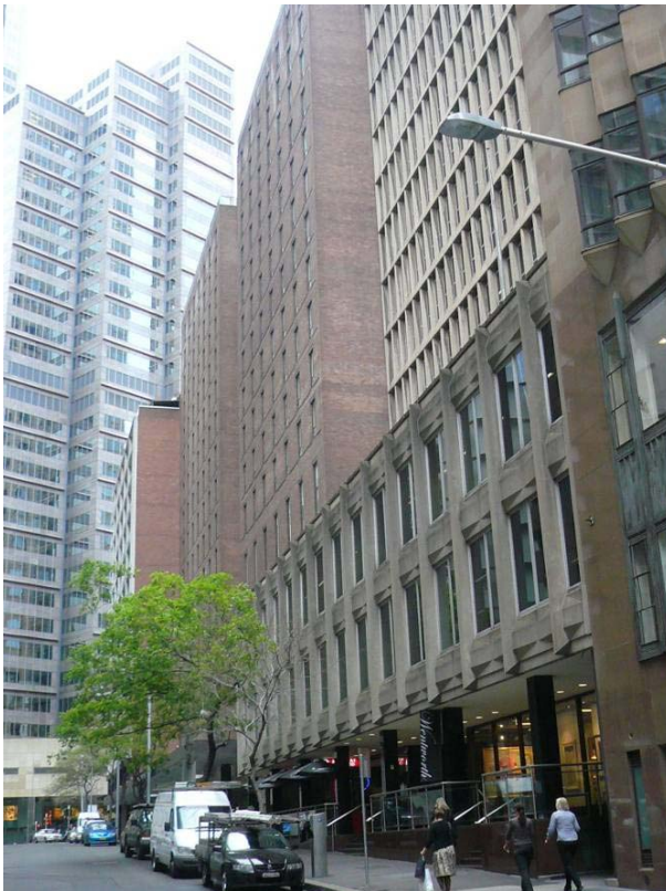
An indication of how the 1970s office building on the opposite side of Bligh Street has adopted the massing model of a lower podium before the tower component.
