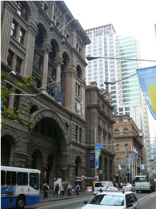
A view down George Street to the General Post Office. These large, late 19 th century institutional buildings add a distinctive and robust character to the precinct that comfortably sits in juxtaposition with the taller modern buildings behind.
