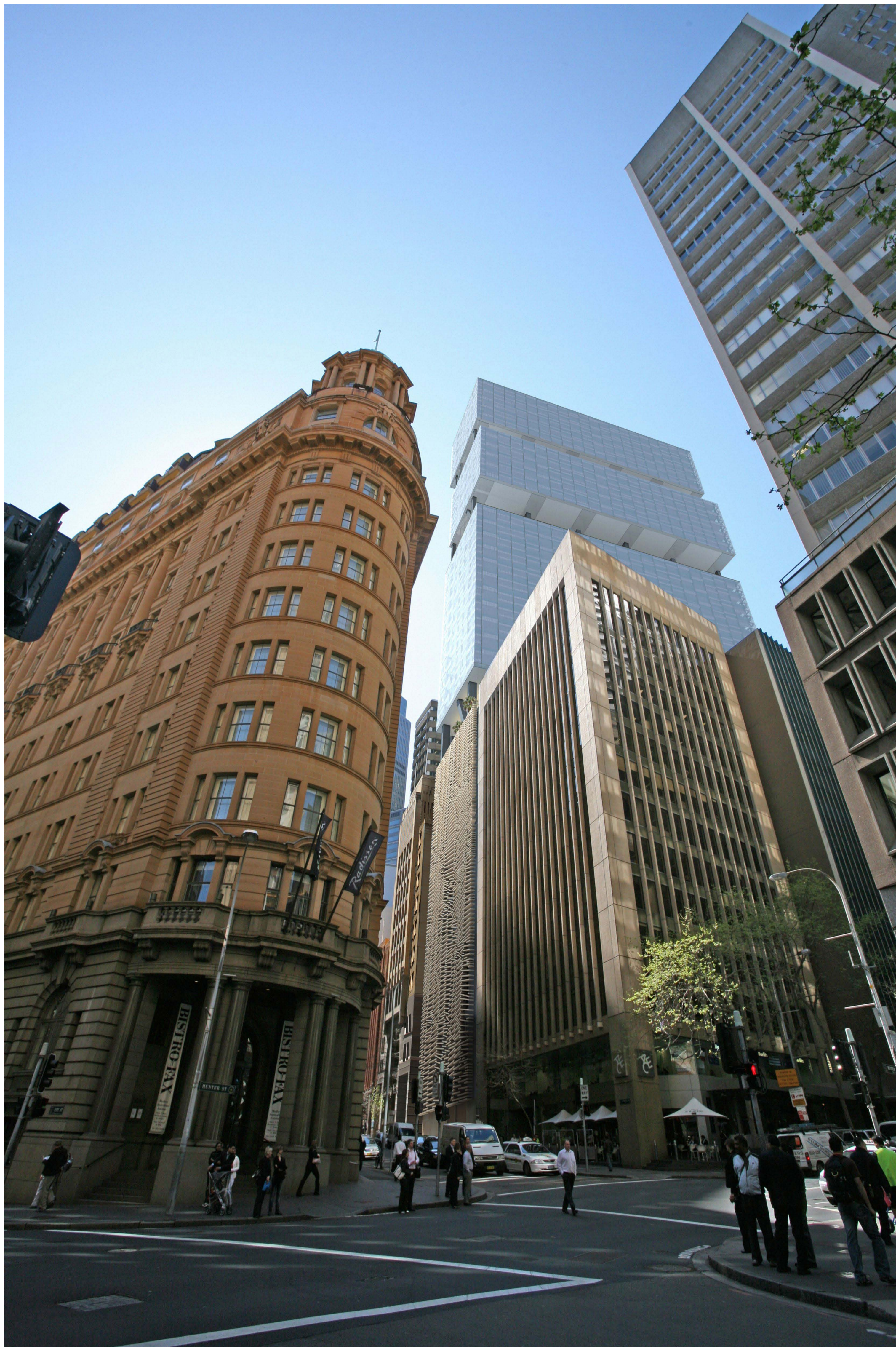
O'Connell Street - Looking From South-West Sculptural wall shown indicatively only. Refer to architectural elevations.
