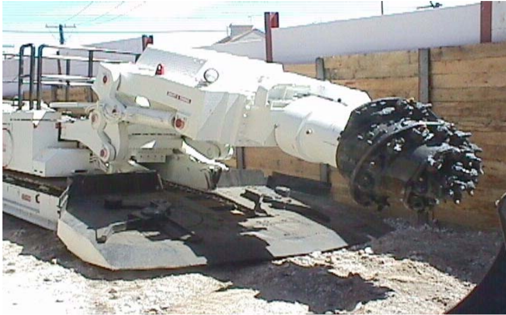
Figure 7-2 Roadheader Tunnelling Operations
