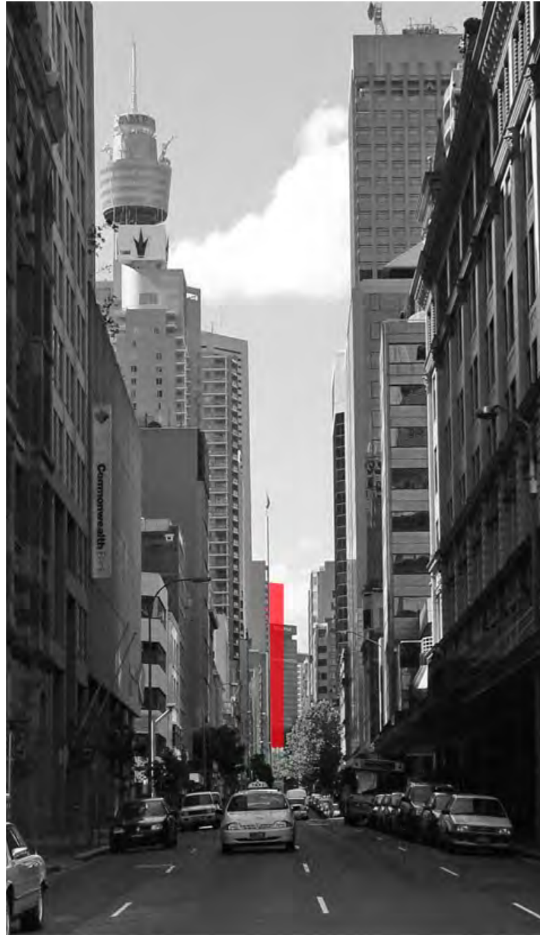
View along Castlereagh Street
