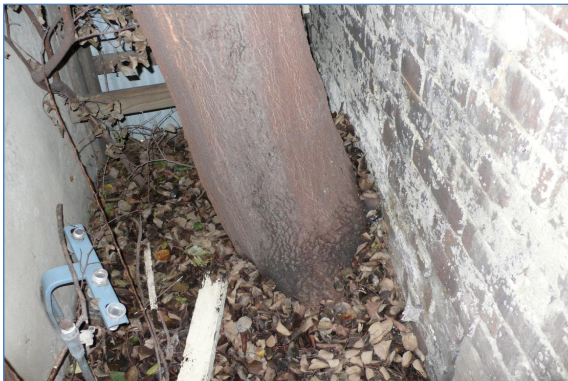
Photo D: Tree 4 adjacent wall of No. 28.
