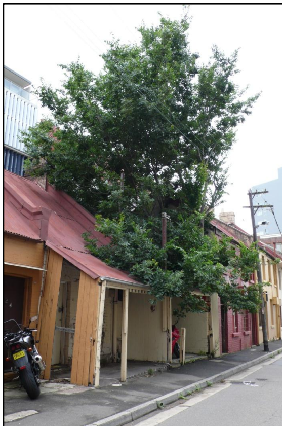
Photo C: Tree 4 Chinese Hackberry, in narrow easement between No. 28 and No. 30-32 Kensington St. Given likely damage to building to be retained this tree is to be removed.
