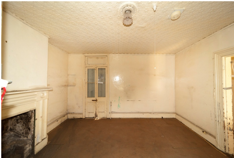
Figure 194. 48 Kensington Street Main front room: looking east. (photo Nat Hughes)
