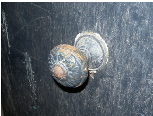
Figure 191. Detail of original door hardware
