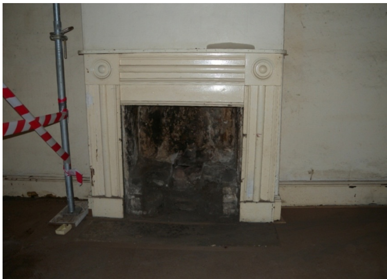
Figure 200. 48 Kensington Street Mid-Victorian fireplace and mantle.
