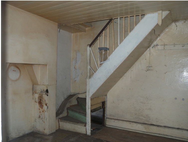
Figure 196. 48 Kensington Street Stair to the upper level.
