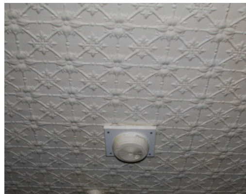
Figure 192. Detail of pressed metal ceiling.
