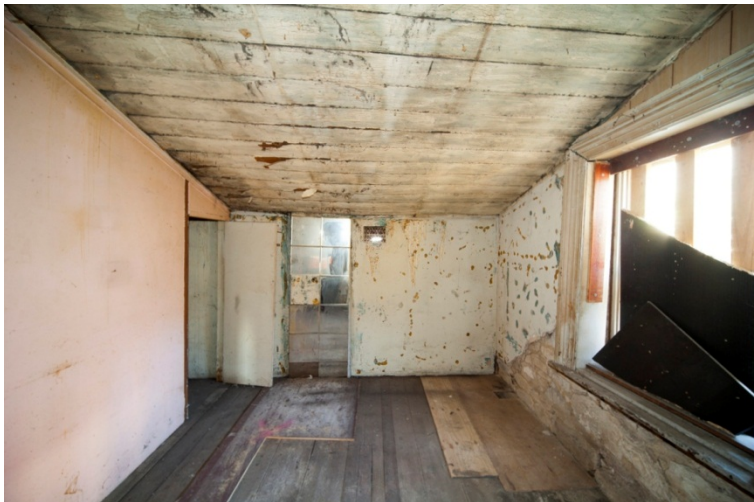
Figure 190. 46 Kensington Street. First floor front room. The upper level of 46 is more intact than the lower. (photo Nat Hughes)
