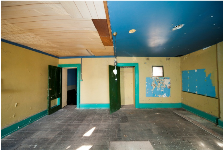
Figure 186. 46 Kensington Street. First floor looking to the rear rooms. (photo Nat Hughes)
