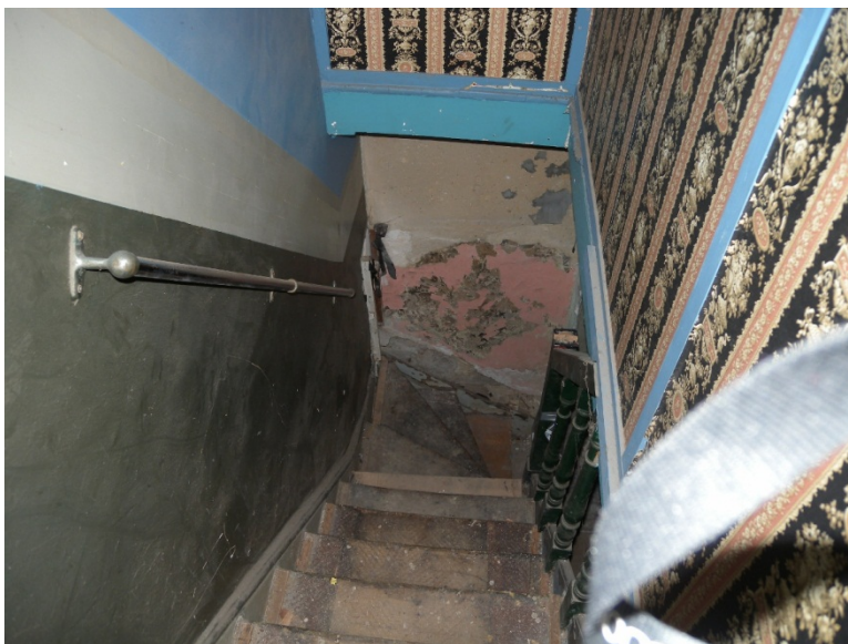
Figure 188. 46 Kensington Street. Detail of stair. Like all of the original terraces in the Kensington Street Precinct the stair is narrow and steep with winders. A steel handrail has been added. (photo Nat Hughes)
