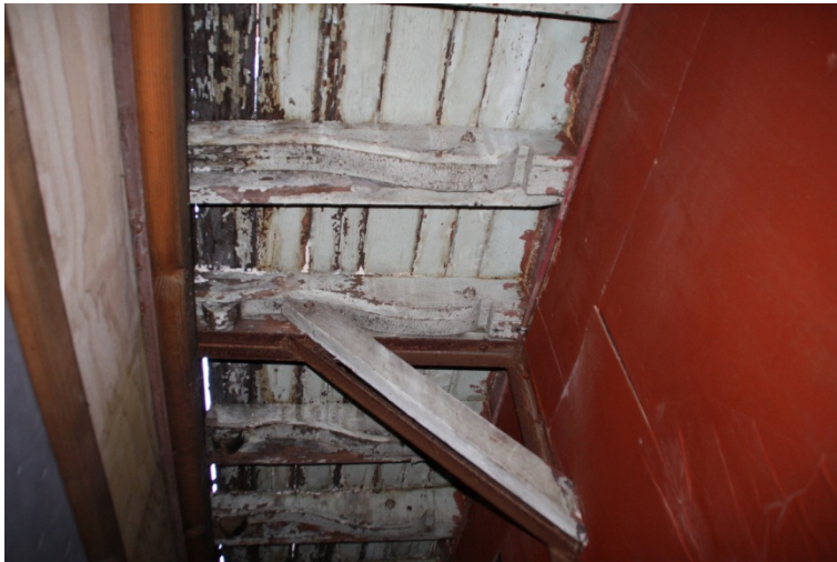
Figure 184. Detail of underside of balcony brackets.
