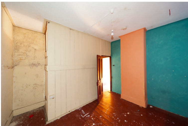
Figure 172. The rooms to the upper level have retained original timber dividing walls enclosing the stair. The alcove on the left is illuminated by borrowed light from a small window above the stair.
