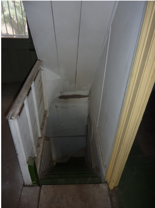
Figure 165. Looking from level 1 to the ground floor. The stairs are pitched steeply.
