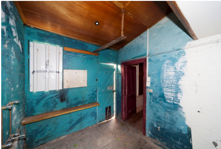
Figure 171. The former service room is under the skillion roofed wing. It has been partially re-lined, but the majority of fabric is original.
