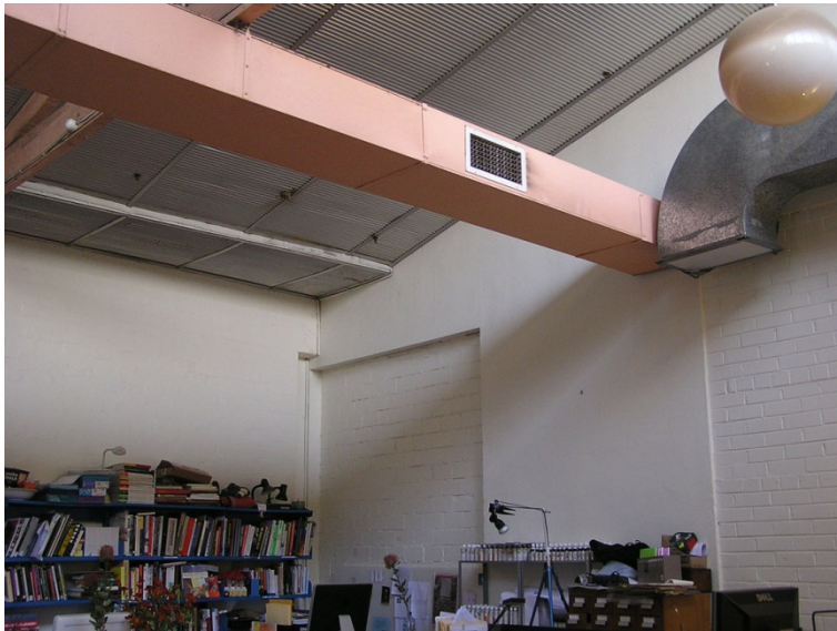
Figure 178. The northern area is of late, and even more basic construction, with rendered walls broken by brick-lined bays with a ripple-iron ceiling.
