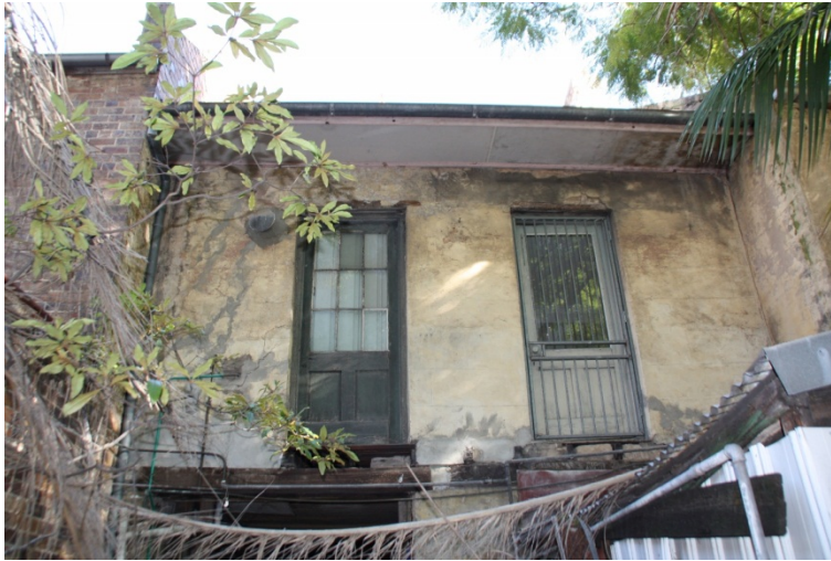
Figure 164. Detail of the upper level rear elevation. Note cut-off joists suggesting that the doors opened onto a rear balcony.
