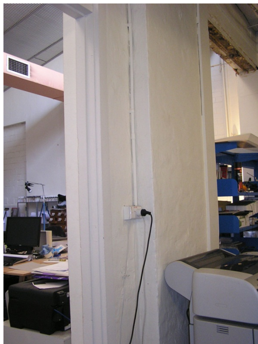
Figure 179. Detail of the wall dividing the northern and southern sections of the building. The wall was originally the external wall of the earlier form of the factory and has been extended through the window and door openings in each structural bay.
