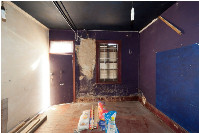
Figure 168. Looking to the front door. Note exposed electrical conduits. Most joinery is original.
