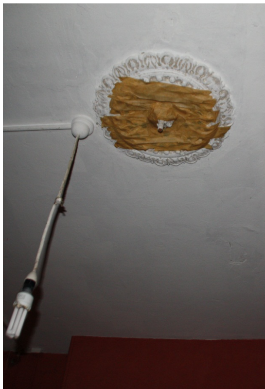
Figure 174. The original central gas fitting has survived in the centre of the ceiling, with adjacent electrical wiring and contemporary low-energy fitting.
