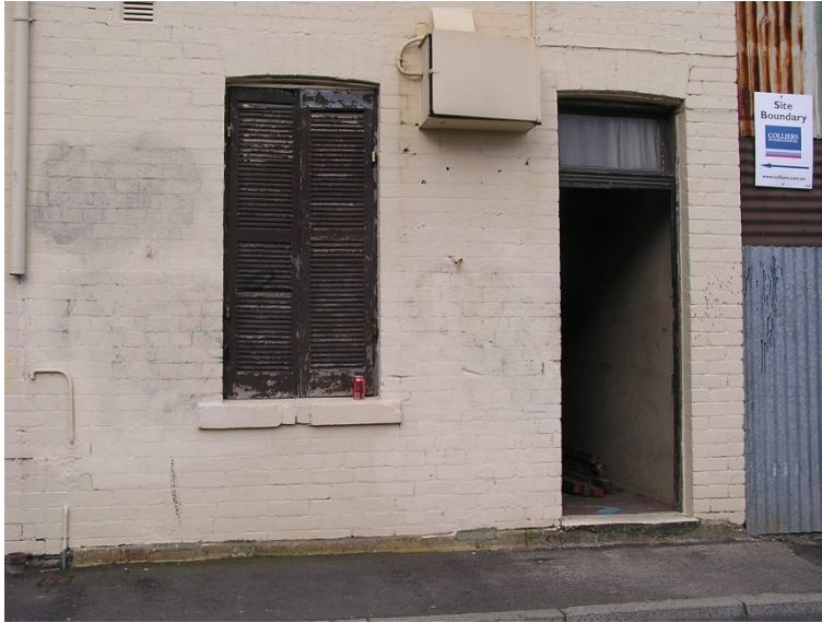
Figure 167. Detail of shutter to window at ground level.
