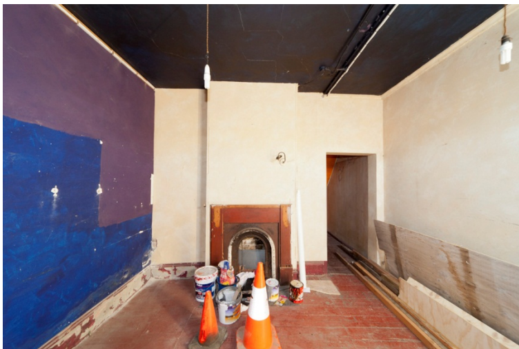
Figure 169. The fireplace is located on the internal wall and rises to the chimney on the ridgeline.
