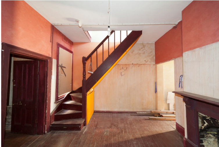
Figure 170. The rear room on the ground floor shares the central chimney. The winding stair is original.
