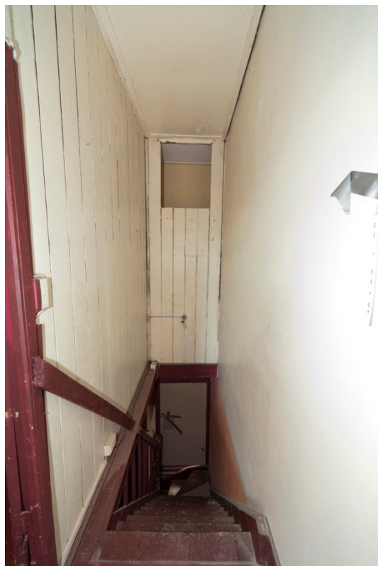
Figure 173. Detail of the stair showing the small opening to admit borrowed light to the alcove behind the stair
