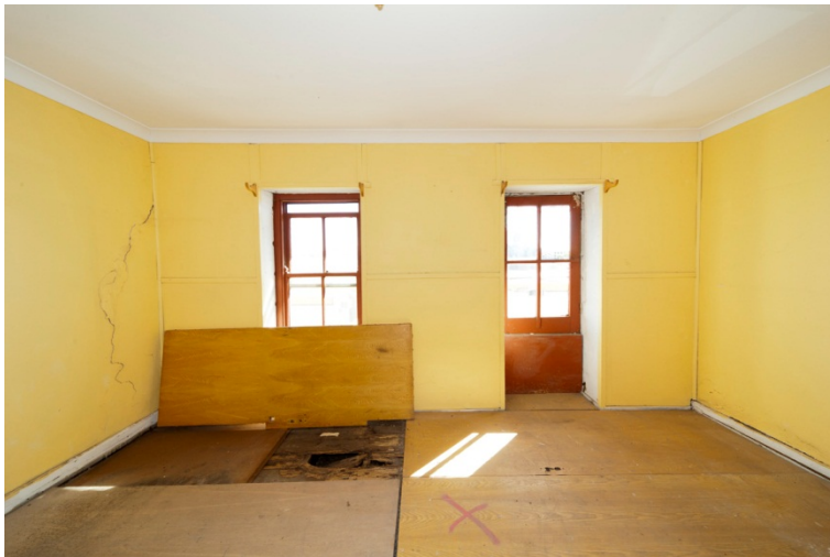
Figure 162. Main upper level room. Note the full-length opening to the window on the right, suggesting that it was formerly a door to a verandah. The window on the left has evidence of an earlier window seat in the bay.
