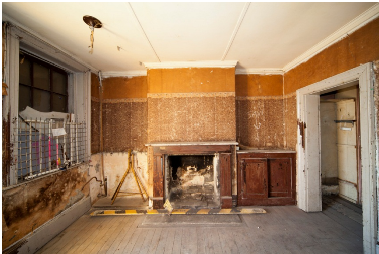
Figure 146. 36 Kensington Street This terrace has retained its early 20 th Century decoration with patterned wallpaper to picture rail height finished by a decorative border, and then a toned pattern above. The original mantle and an early side cupboard have also survived. The ceilings have been replaced. (Photo: Nat Hughes)
