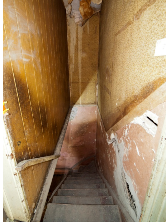
Figure 150. 36 Kensington Street Looking down the stairwell. (Photo: Nat Hughes)
