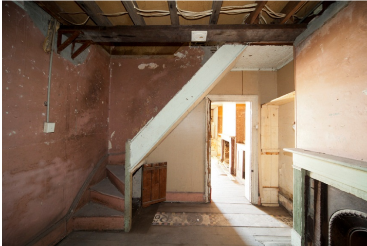
Figure 148. 36 Kensington Street The stair to the bedroom floor is accessed from this room. Joinery to this back room is simpler, although elements such as the fire grate and timber mantle have survived in both rooms. The ceiling and cornices have also been removed from this room. (Photo: Nat Hughes)
