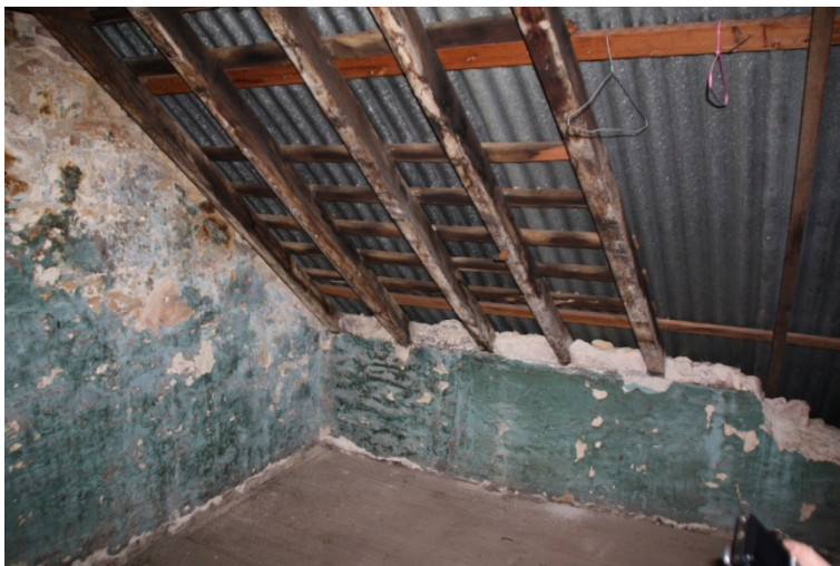
Figure 163. The roof framing has been partially replaced but evidence of the earlier dormer windows can still be seen in the open area to the right of this image.
