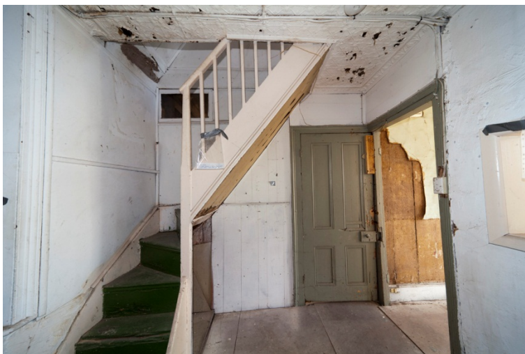
Figure 160. The stair to the upper level is steep with winders. The stair rail is original.
