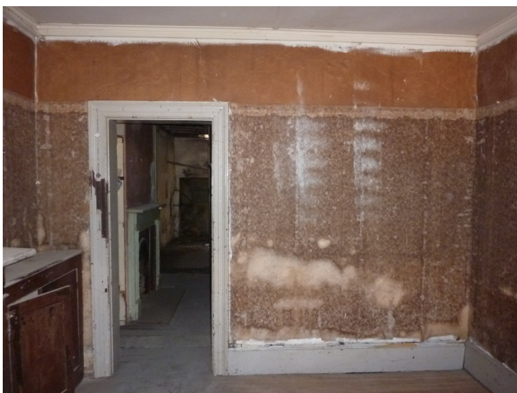
Figure 147. 36 Kensington Street Looking to the back room from the front window.
