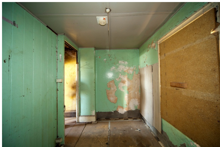
Figure 153. 36 Kensington Street Back room to Level 1 (Photo: Nat Hughes)
