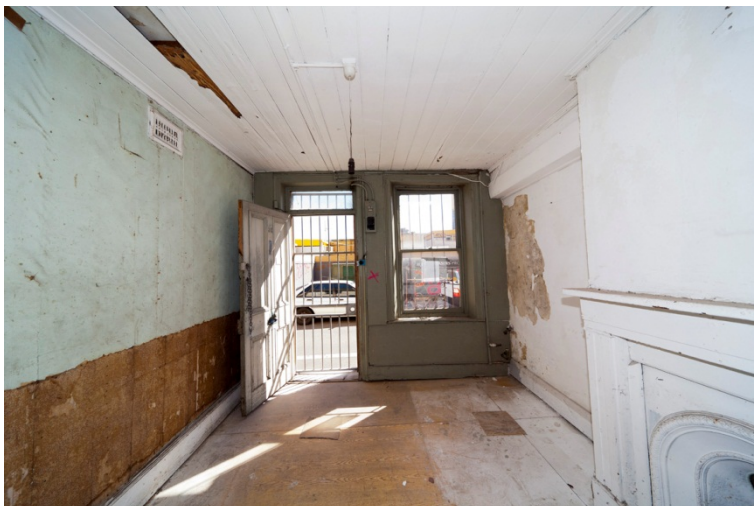
Figure 157. Looking to the front door. The wall on the left of the room is the timber dividing wall to the carriage drive-through (photo: Nat Hughes).
