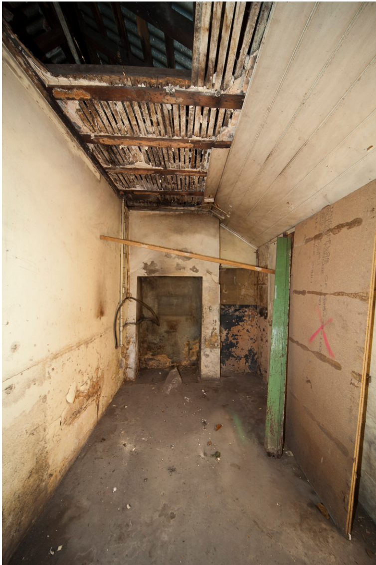
Figure 152. 36 Kensington Street — kitchen area at the eastern end of the gabled wing.
