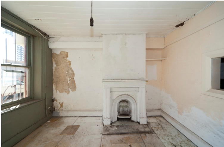
Figure 158. Ground floor: painted mid-Victorian timber mantelpiece with cast iron fireplace to front room chimney breast, timber tongue and groove board ceiling. The second room on the upper level also has a pressed-metal ceiling.
