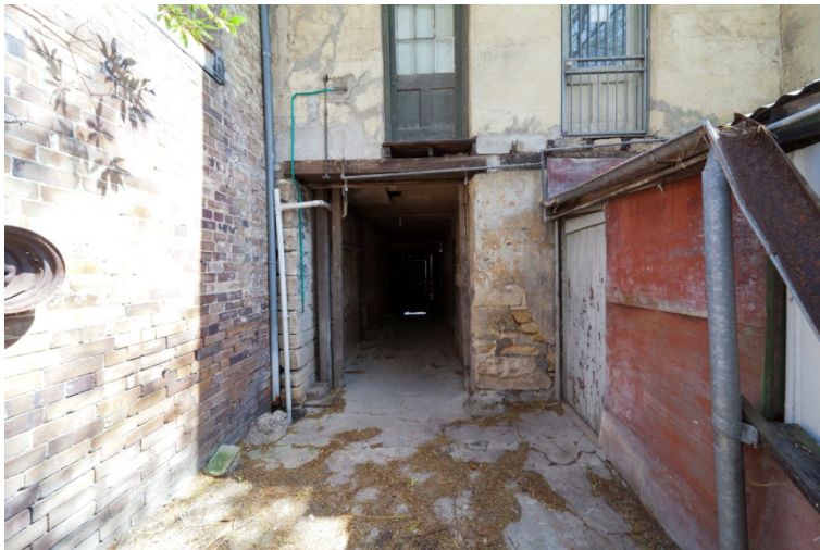
Figure 156. Rear of building showing the access to the street. No evidence of the stable described in the Sands Directory remains.
