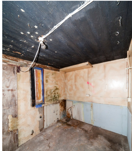
Figure 130. 30 Kensington Street: first floor room. (photo: Nat Hughes)
