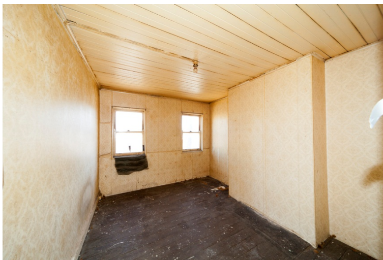
Figure 136. 32 Kensington Street. First floor room with stair enclosure. (photo: Nat Hughes)
