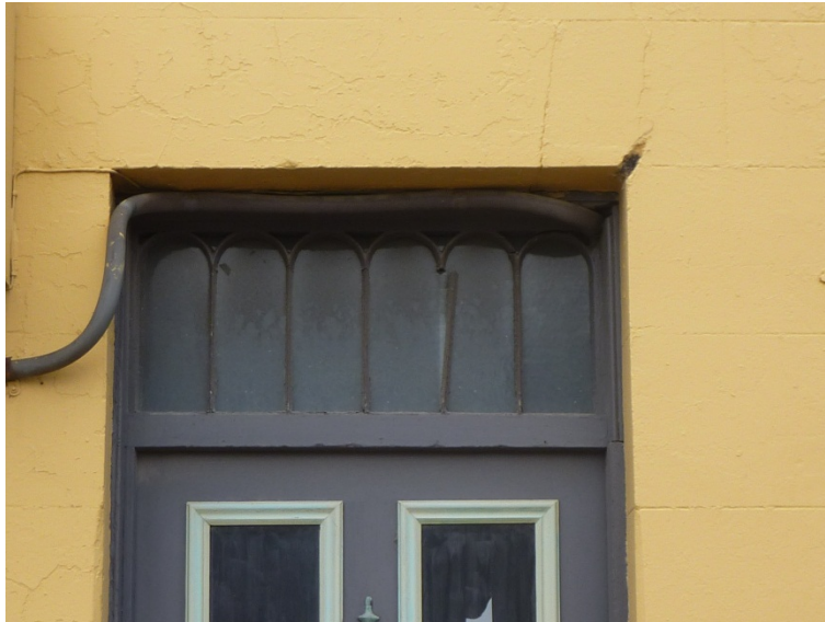
Figure 137. 34 Kensington Street Delicate arched detailing has been applied to the fanlight glazing.
