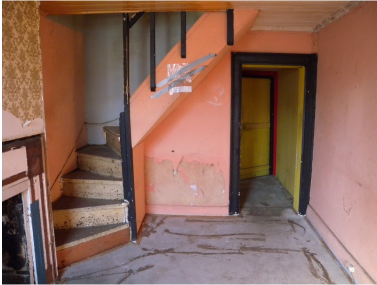
Figure 132. 32 Kensington Street: main room and stair.
