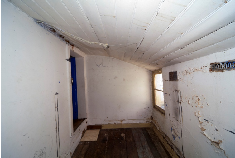
Figure 128. Upper level at rear – under roof 30 Kensington Street (photo: Nat Hughes)
