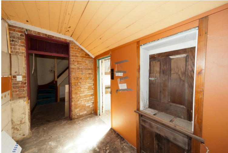
Figure 142. 34 Kensington Street Taken from the kitchen wing looking to the main house. (Photo: Nat Hughes)
