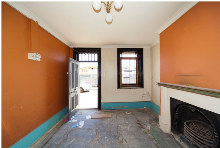
Figure 138. 34 Kensington Street Main room. One of the indicators of the modest scale of these terraces, like most along Kensington Street, is revealed by the front door opening directly into the main living room with no hall or reception room. This terrace has been painted in the relatively recent past.
