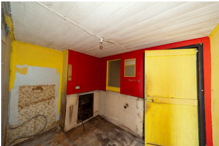
Figure 134. 32 Kensington Street: kitchen (photo: Nat Hughes)
