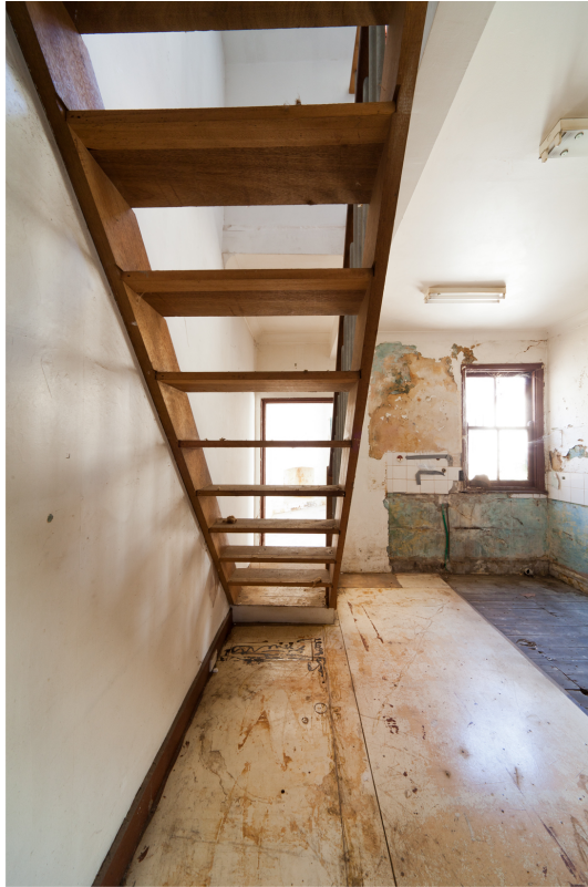
Figure 113. No.26: The ladder-like stair has been replaced by a wider and easier to negotiate stair. (Photo Nat Hughes)
