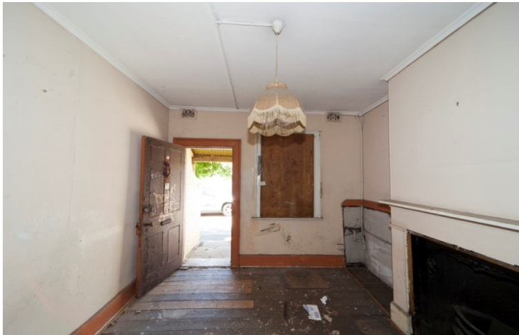
Figure 117. No.28: main room. Note electrical conduit to protect wiring and the simple and original mantle over the fireplace. (Photo Nat Hughes)
