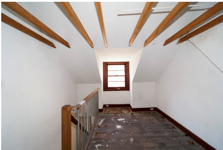
Figure 115. No.26 the attic space has also been refurbished with the ceiling beams retained as a feature. The new window is wider than the original, leading to impact on the rhythmical qualities of the roofscape of the group. (Photo Nat Hughes)
