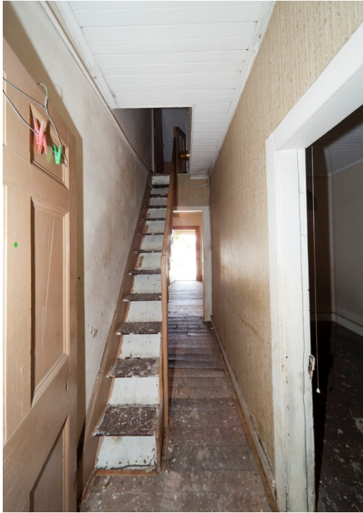
Figure 119. No.28: This terrace is very intact and has retained much of its original detailing including the narrow hall with ladder-like stair to the attic level. (Photo Nat Hughes)
