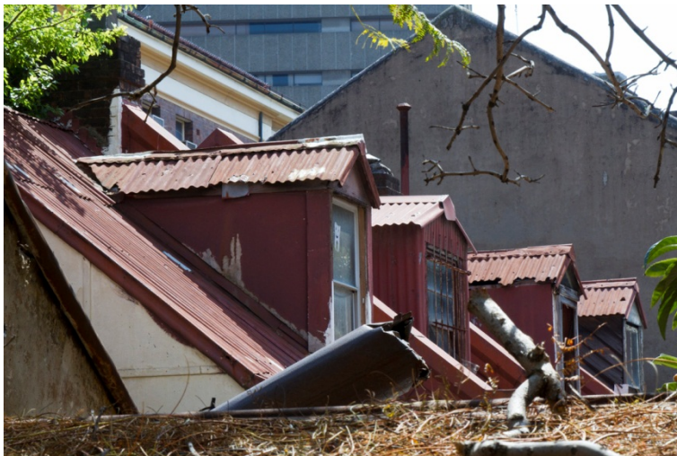
Figure 92. Detail of the dormer windows.
