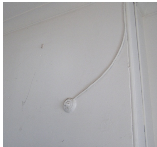
Figure 96. The simple electrical wiring is fixed to the walls. Many of the fittings are intact.
