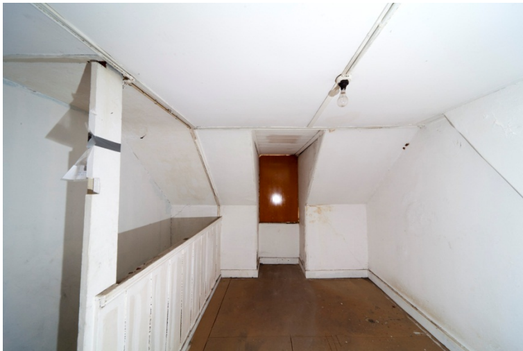
Figure 104. No.22: attic space (photo: Nat Hughes)
