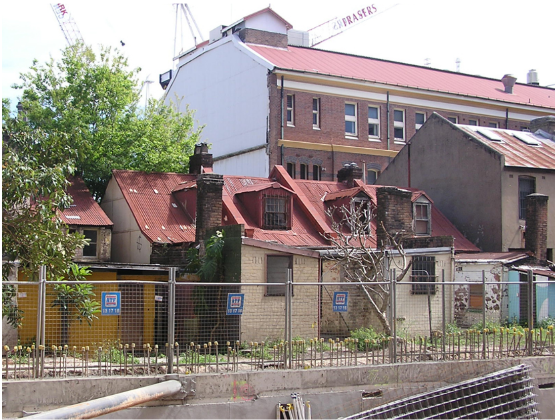
Figure 91. Each of the four terraces feature a timber clad gabled dormer window to the rear roof plane. The dormer to No.26 (second from the left) has been enlarged and clad in corrugated steel.
