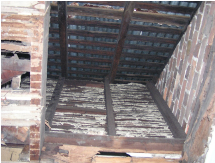
Figure 100. No.22: showing narrowness of stair to fit into standard hall space. Plus note the exposed lathes to upper level – missing plaster
