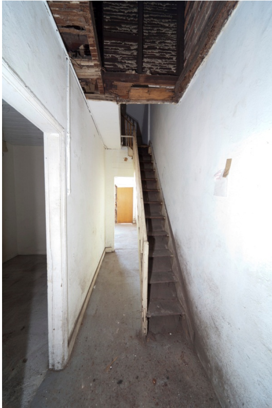
Figure 100. No.22: showing narrowness of stair to fit into standard hall space. Plus note the exposed lathes to upper level – missing plaster
