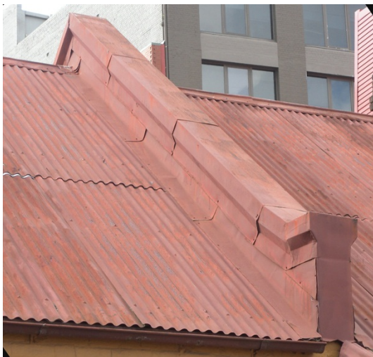
Figure 95. Detail of the capping to the party walls between the terraces.
