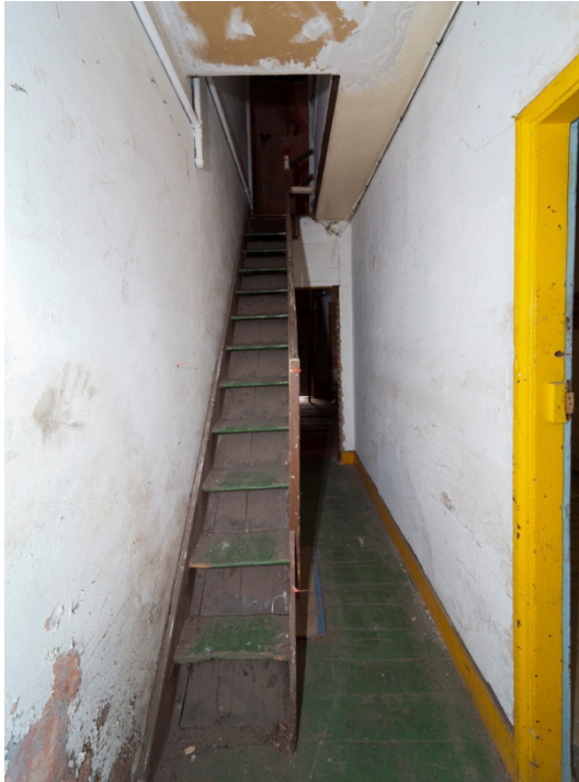
Figure 108. No.24: hall and stair. (photo: Nat Hughes)
