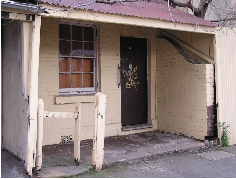
Figure 93. The terrace at 28 Kensington Street is the most intact of the group, with remnants of the fence and gate extant. Note the worn threshold under the gate.
