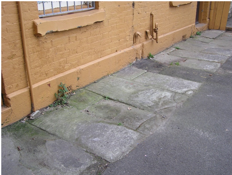
Figure 94. The flagging to the original verandah floor of the terraces 22 and 24 Kensington Street has been exposed by the removal of their roof.
