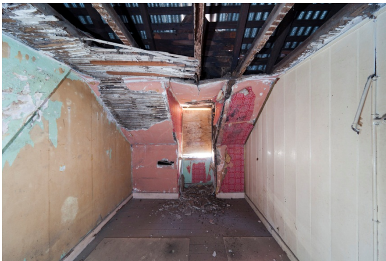
Figure 110. No. 24: attic space (Photo Nat Hughes)
