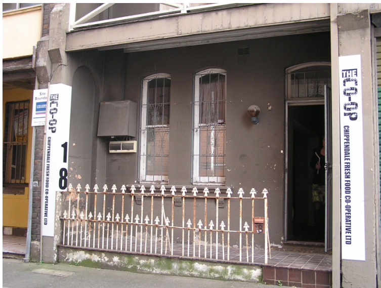
Figure 81. Detail showing veranda area. The cast iron palisade fence is original, although the tips of the decorative heads have been trimmed..
