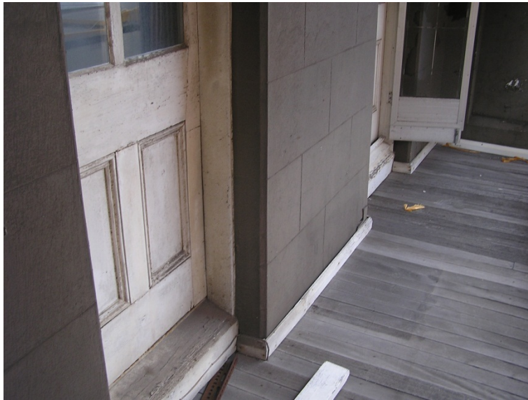
Figure 89. The floor to the verandah on the upper level is hardwood and is in very good condition, suggesting that it may have been replaced, or that the verandah was infilled for at least part of the time since its construction.
