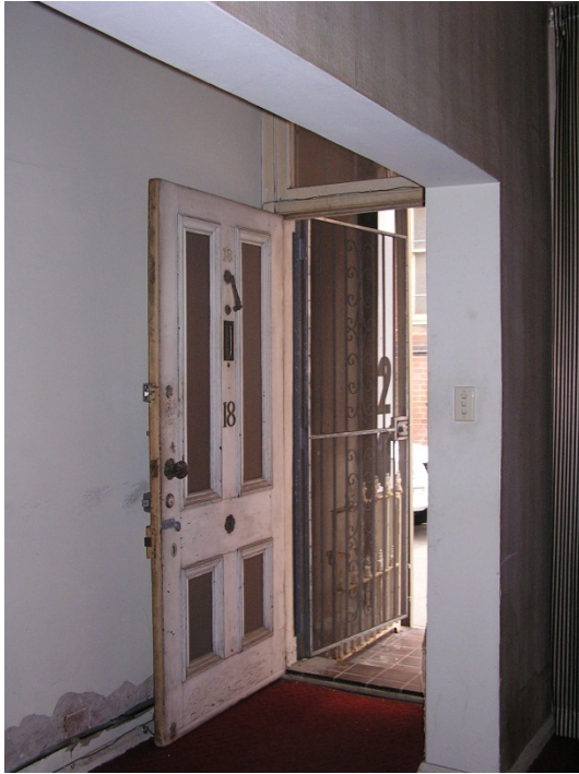
Figure 86. (Left) Looking toward the front door showing one of the larger openings that have been cut into the internal walls
