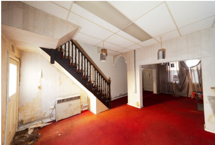
Figure 83. The interior spaces have undergone significant alteration to provide office-style accommodation. The lower level has been altered by removal of the wall dividing the main room and the hall. Circa 1970s acoustic panel ceilings have been installed throughout the terrace. Architraves to internal doors and skirting boards are modern, floors are carpeted, and walls are generally wallpapered. There is evidence of original plaster ceilings above the acoustic panel ceilings. Internal doors are modern hollow-core doors. The interior also features circa 1970s shelving and light fittings. (Photo: Nat Hughes)
