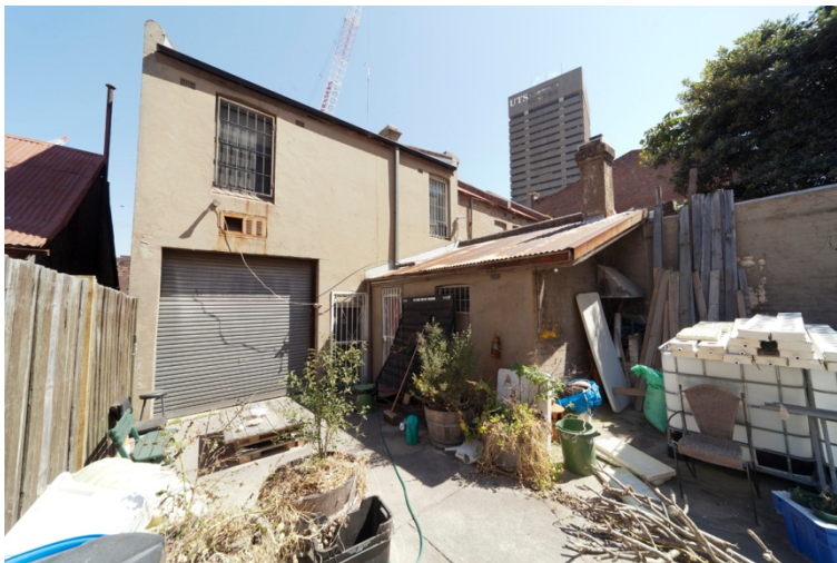
Figure 85. The rear elevation has been cement rendered. Its elevation is simple, with two windows to the upper level and a small skillion roofed extension wing. Two skylights have been inserted in the main roof pitch. Evidence of recent modification includes the opening created to install an air-conditioning unit at some time in the past.
