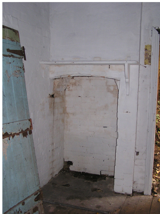
Figure 77. The original kitchen hearth and ledged back door are in the rear room. No contemporary services are evident.
