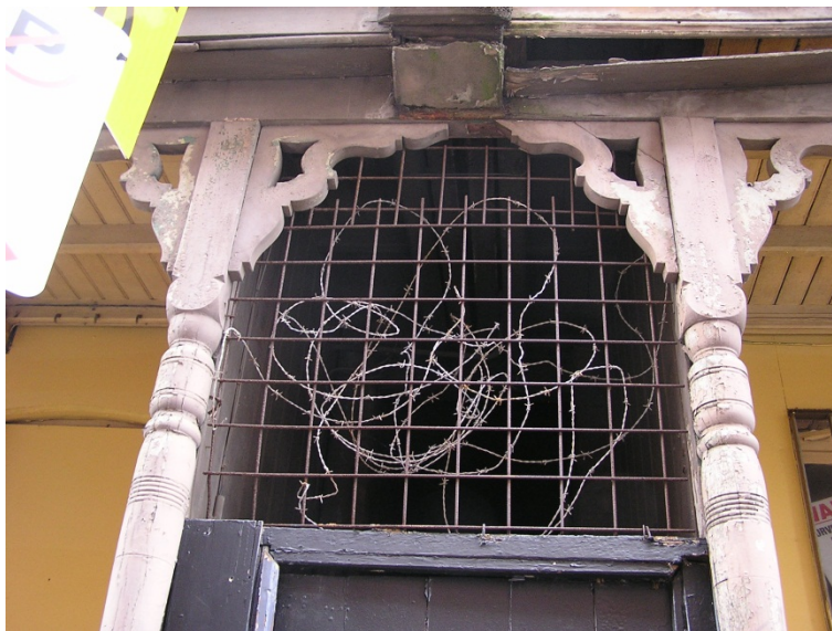
Figure 66. The terraces have a central nightsoil lane, which is flanked by turned timber posts and decorative timber brackets.
