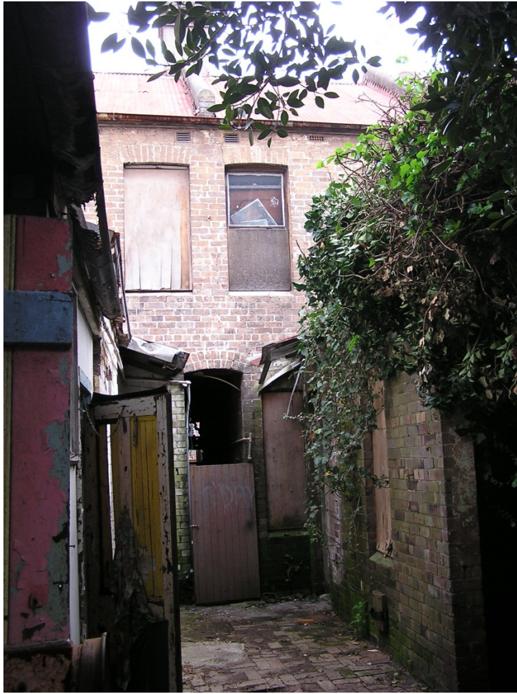
Figure 70. Walls are built of common brickwork, including to walls of the nightsoil passageway. The brickwork to the skillin-roofed wings has been painted to No.16A.
