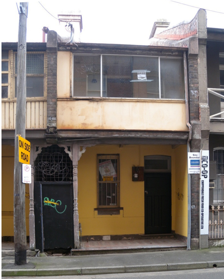
Figure 65. At the first floor level, behind the balcony enclosures, each terrace features a central doorway opening which originally housed a pair of glazed timber French doors (now missing to both), with fanlights above. Both terraces retain the fanlights. The balcony to 16 was used as a bathroom, with evidence of plumbing and venting extant and a solid infill to the street.
