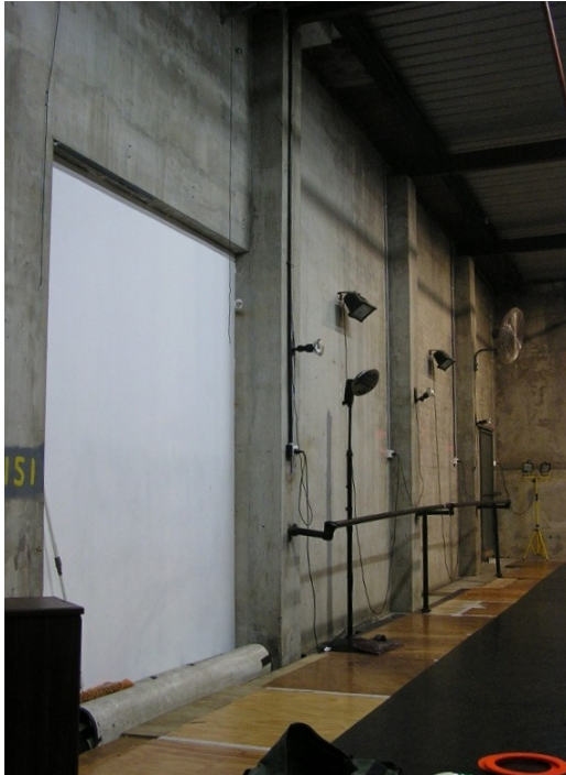
Figure 60. The current use of the building is as a rehearsal space, with timber floor over concrete base with tarquette surface. Barres have been fixed to the northern wall with fans set high on the wall. The opening to 12 Kensington Street has been infilled with lightweight materials and the smaller door covered by a curtain. A door at the eastern end of this wall provides access to the small area behind 12 Kensington Street.
