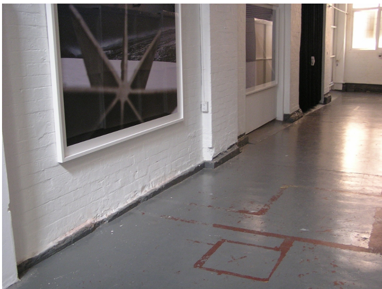
Figure 53. Floor: Floors are simple, formed from a polished/painted concrete slab. Markings indicate former warehouse use. The slab slopes down toward the roller door opening to allow vehicular access to the interior.
