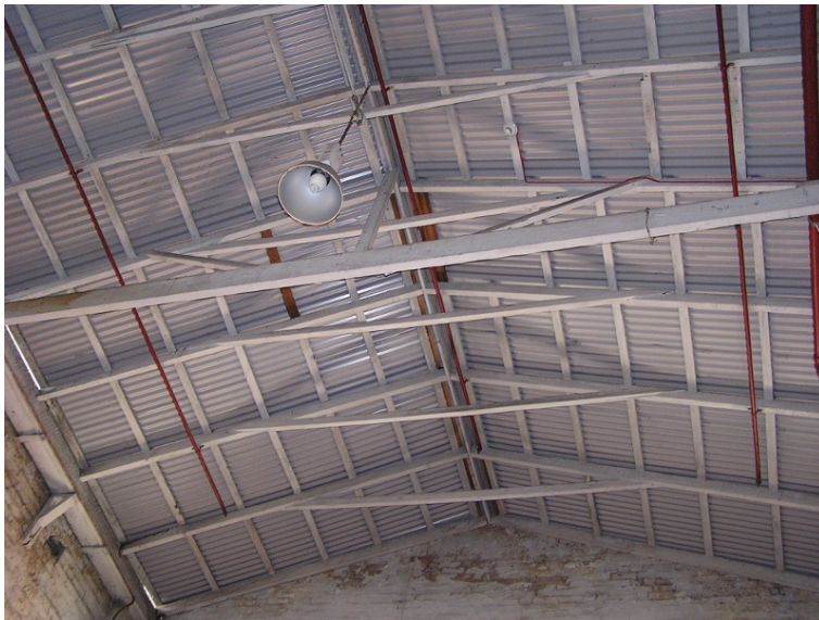
Figure 52. Roof and ceiling The roof of the building is a simple structure with corrugated steel sheeting (non-original) laid on simple timber trusses sitting on wall plate. No ceiling is present.
