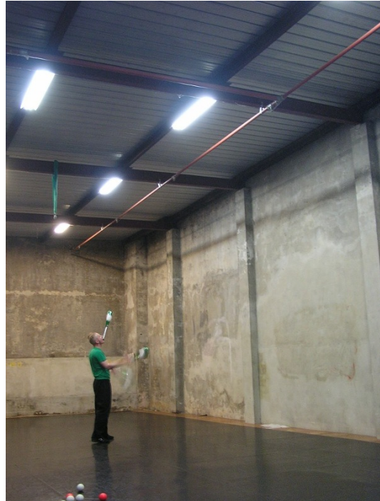
Figure 61. The roof is a simple structure with corrugated steel sheeting (non-original) laid on light timber trusses at a very low pitch. The space has negligible detailing. Walls are rendered in cement – no paint finish. Vehicular licence plate numbers have been painted around the walls – associated with earlier use as garage.
