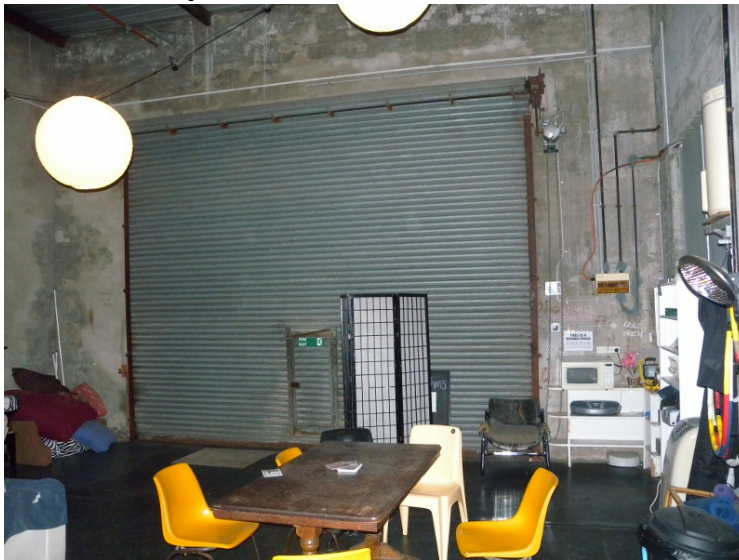
Figure 60. The current use of the building is as a rehearsal space, with timber floor over concrete base with tarquette surface. Barres have been fixed to the northern wall with fans set high on the wall. The opening to 12 Kensington Street has been infilled with lightweight materials and the smaller door covered by a curtain. A door at the eastern end of this wall provides access to the small area behind 12 Kensington Street.
