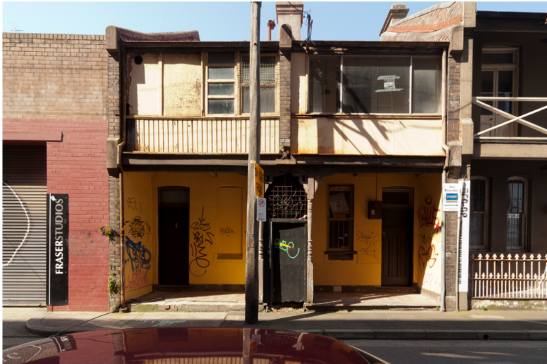
Figure 63. The pair of terraces at 16 and 16A Kensington Street. The face brickwork has been covered by fibre-cement panels but is extant beneath. The upper level verandahs have been enclosed by lightweight materials but the original external elevation to the terrace has survived.
