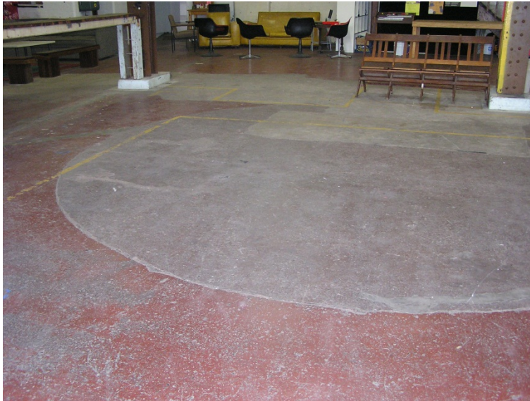
Figure 43. Marking on floor at ground level providing evidence of an earlier vehicular-scaled turntable set into floor (the mechanism has been removed and the area infilled with concrete slab). The position of the turntable does not align with either the door opening or the lift.
