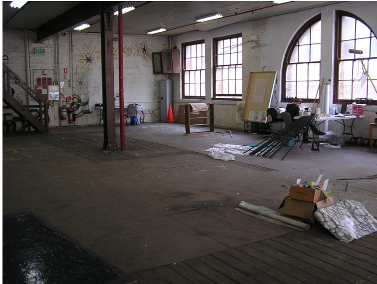
Figure 36. Interior: Level 2 has the same structural configuration as the ground floor with the riveted beams and columns aligned with those below. Arched bays sit along the eastern wall with fittings for gas lanterns built into two of the bays. The lift bay is lined to c1200mm above floor level with heavy steel mesh above. A small sign is attached to the lift doors warning of load capacities in hogsheads. Floors are timber: they are mainly sound, although the scratched surface provides evidence of heavy loads being dragged. Floorboards have been replaced in places. The stair to this level is not meshed or gated.
