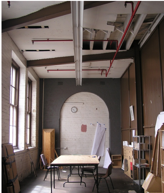
Figure 40. A small office area has been formed on each level between the lift and windows overlooking Dwyer Street. This area is not reinforced and has a ripple iron ceiling lining, and tongue and groove timber lining has been fixed to the wall of the adjacent lift cage.
