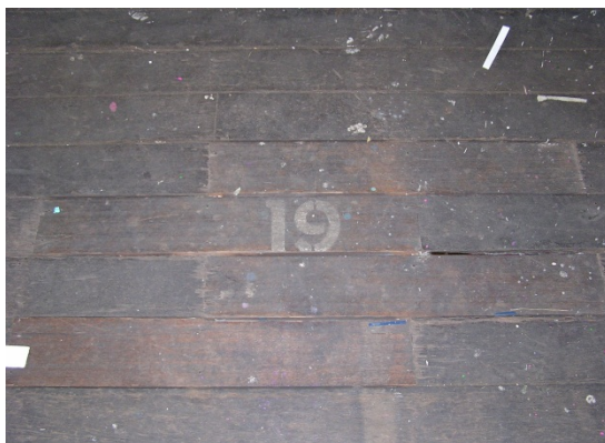
Figure 38. The floor to the ground level is a poured concrete slab with a separate poured slab where a turntable was previously located (note that this was offset to the door openings). There is also small area of patching near Dwyer street. The floors to the upper levels are timber tongue and groove boards — mostly intact, but patched in places. Neatly painted numbers survive to the storage areas on the upper floors. The boards throughout are worn, providing evidence of the use of the space; but appear to be sound.
