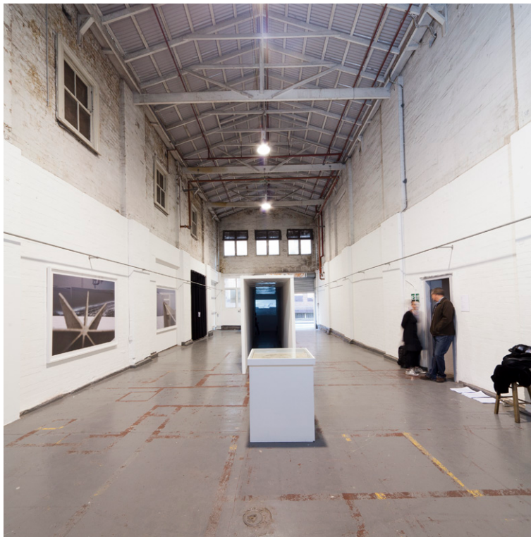
Figure 50. The interior of the building has been gutted, including the removal of the upper level, to create a single large space. Door openings have been cut in the walls to the north and south to provide direct access between the three buildings by the Brewery. (Photo: Nat Hughes)
