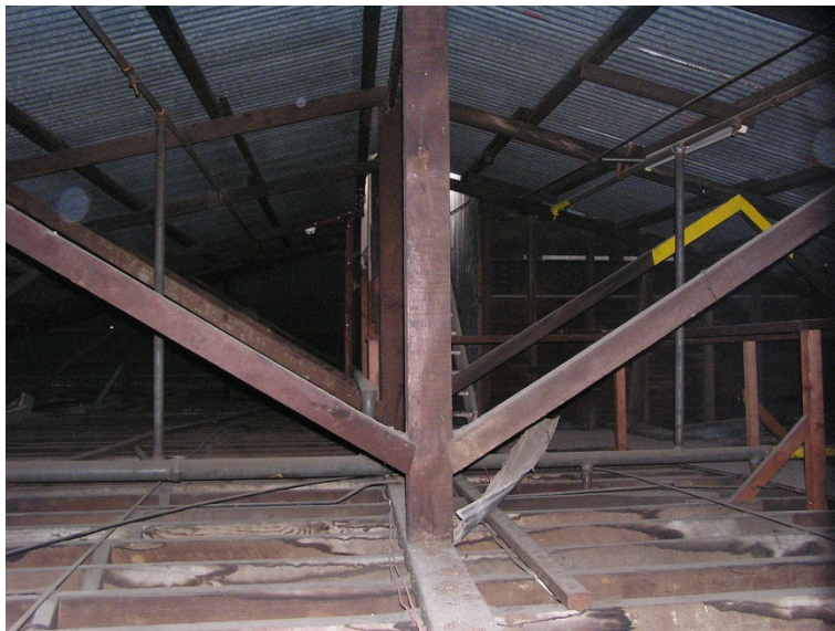
Figure 37. Within the roof space. A simple king post truss timber construction with corrugated iron sheeting. A timber walkway provides access to the roof exterior and the lift motor room.
