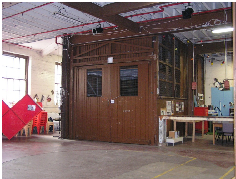
Figure 40. A small office area has been formed on each level between the lift and windows overlooking Dwyer Street. This area is not reinforced and has a ripple iron ceiling lining, and tongue and groove timber lining has been fixed to the wall of the adjacent lift cage.
