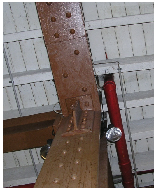
Figure 41. Looking up to the underside of the floor above showing riveted steel girder construction.
