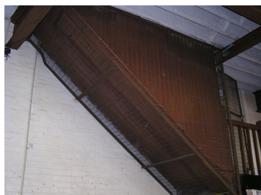
Figure 39. Staircases are banked on the southern wall, although the configuration varies between floors. All are open timber tread, but evidence such as grille doors and caging provides evidence of use as secure (bonded) storage area. The stair between ground and first floors is open tread and rail to a mid-way landing, and fully enclosed (with timber boarding and welded mesh overlay) to the upper part. Evidence of heavy grille (likely to be fixed or possibly a gate) to the stair (a lighter gate with welded mesh is extant).
