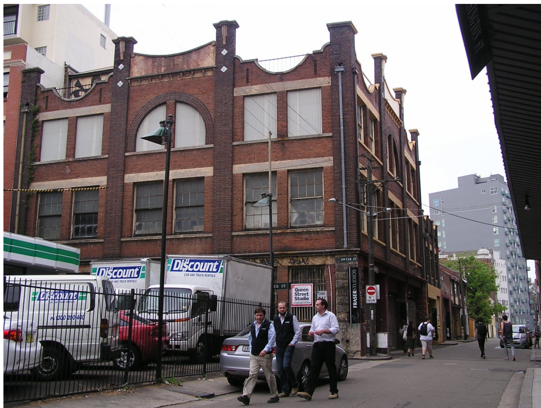
Figure 23. Former Motor Garage and Rum Cask Store at 2-10 Kensington Street viewed from the north (Broadway).
