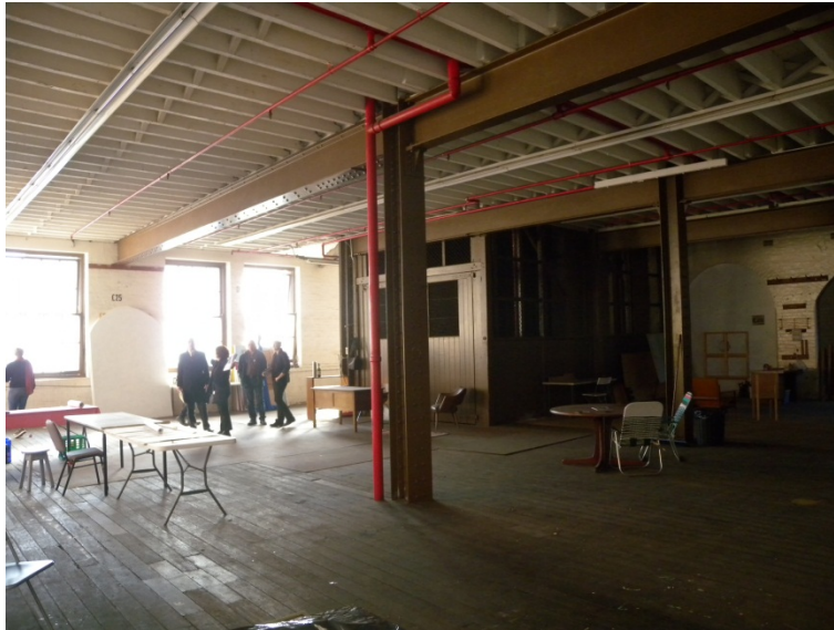
Figure 33. Interior – structural details. The structural capacity of the building was improved in the 1930s by the addition of Dorman and Long 'I' beams and columns in order to carry heavier loads as part of its use as a Bonded Store for alcohol. The main part of the internal structure is now supported by steel columns and beams framed by riveted girders, with the original lighter weight supports to the administration areas.
