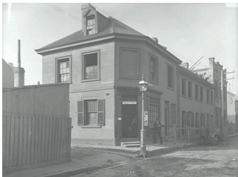
Figure 24. The corner of Dwyer and Kensington Streets c1908 prior to demolition for construction of the Motor Garage/Rum Bond Store on the corner in 1913. The newly built warehouse at number 12 is visible behind. (Sydney City Council Archives image Pix005-005108)
