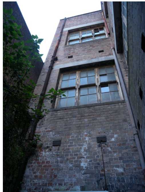
Figure 30 (above): The building is built to the eastern and southern boundaries with the exception of a small light well set at the south-eastern corner of the property. It is accessed only via a door at ground level. Large timber framed windows open to the well on each level.
