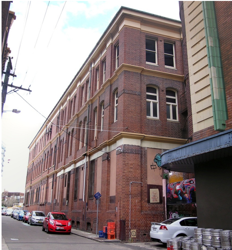
Figure 21. The former Administration Building forms an important edge to the Kensington Street Precinct due to its imposing scale and strong patterning created by the rhythms of the fenestration, the projecting mouldings that direct the eye along the street and the physical barrier it provides between Kensington Street and the interior of the main Brewery Precinct.
