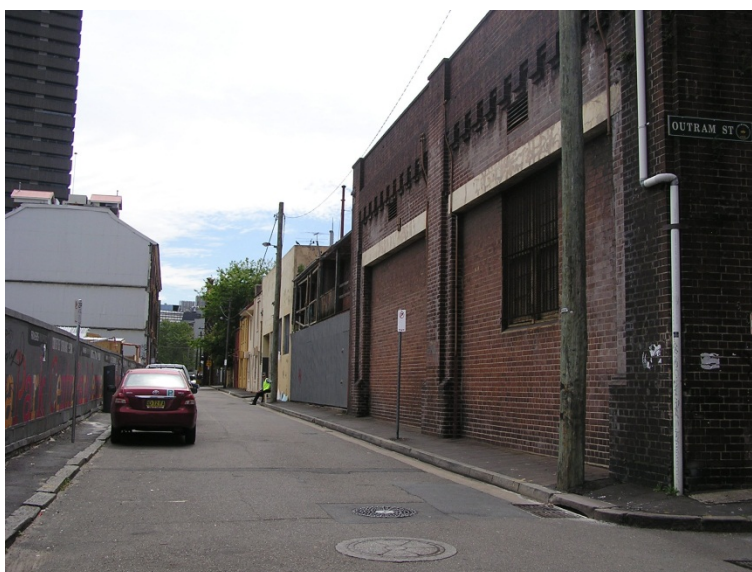
Figure 20. View towards Broadway from the southern end of the Precinct (Outram Street). The character of the streetscape at this end is more strongly industrial, being created by the Brewery's former Motor Garage on the corner and the white infill factory (42-44) in the middle distance of this photo; and is reinforced by the featureless hoarding protecting the sandstone terraces at 46-48 Kensington Street.
