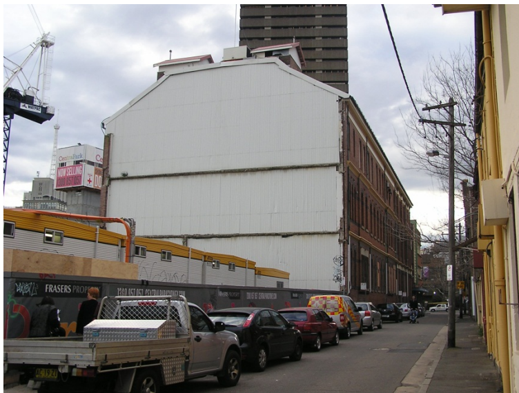
Figure 22. Southern elevation of the Administration Building showing the temporary wall erected to protect the Administration Building following the demolition of the earlier extension. High rise development associated with Central Park is under construction in the area to the left of this photo. This building will change both the scale and movement patterns between the Kensington Street Precinct and the adjacent Central Park.
