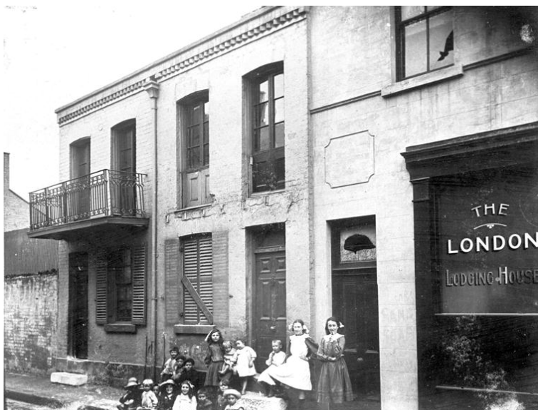
Figure 7. The London Lodging House was demolished to allow construction of the Aerated Waters Factory (now part of the Administration Building on the main brewery site).
