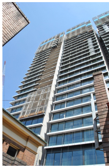
Figure 27. The Kensington Street Precinct is located within an area undergoing rapid and visually dramatic transformation, with the UTS building (L) now being challenged by the height of the buildings under construction within the Central Park redevelopment (R).
