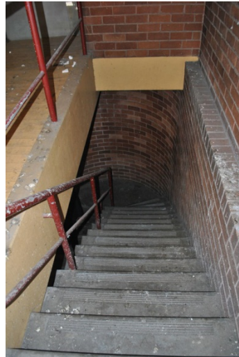
Figure 99. Looking into the lightwell from the roof terrace. Note the skylight to the saloon bar that is now blocked
