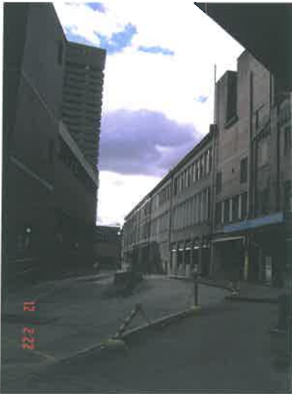
Figure 33 - Main Avenue (former Kent Road) looking north from the former Kent Brewery Yard showing the continuous run of the administration buildings on the right
