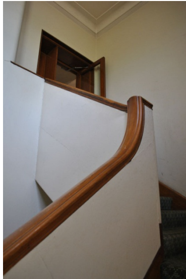
Figure 89. Decorative elements include niches placed regularly up the stair fitted with simple semi-cylindrical lights.
