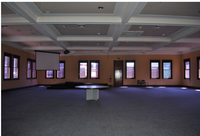
Figure 72. Most of Level 2 has been stripped and converted to a large open plan office.
