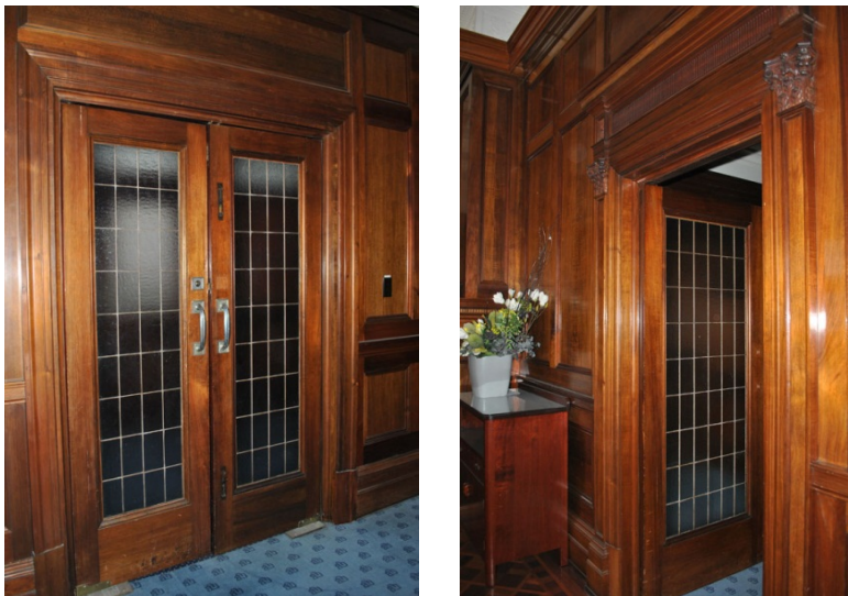
Figure 58. Doors to the Ante Room.
