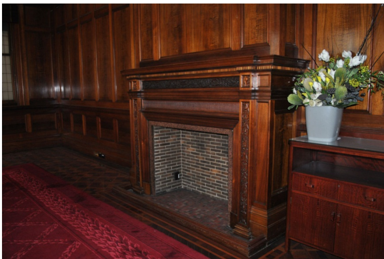
Figure 61. The original fireplace with miniature brick lining and carved timber surround.
