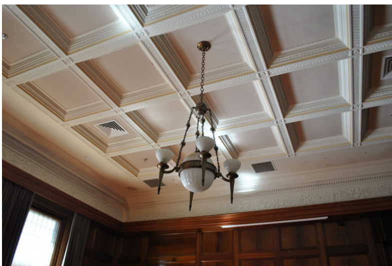
Figure 66. Detail of the ceiling of the Boardroom.
