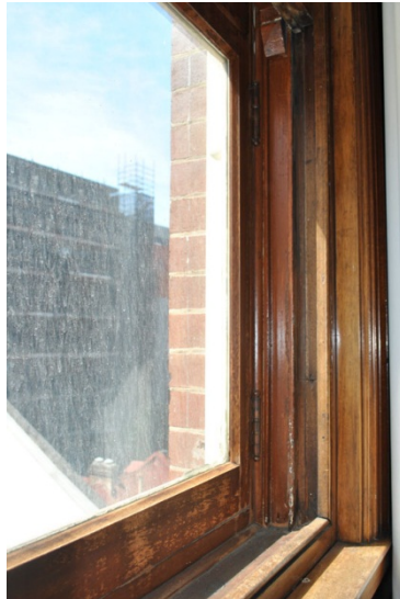
Figure 64. and 65. The windows to the Boardroom are double-glazed sash windows set into separately operable tracks.
