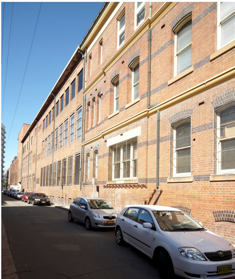
Figure 31. The western side of Kensington Street was dominated by the 3-4 storey scale of the brewery buildings that lined it and dwarfed the adjacent terraces on the eastern side. This photograph was taken prior to the demolition of most of the structures on the site. The building in the middle distance is the later extension to the Administration Building which has now been demolished.
