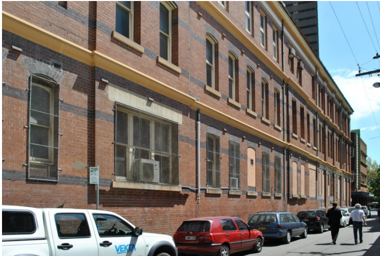
Figure 30. The Administration Building forms an important edge to the northern end of Kensington Street due to its imposing scale and strong patterning created by the rhythms of the fenestration and projecting moulding which direct the eye along the street. The building is also notable for its lack of access from the public domain, reinforcing the prominence in the streetscape. Although the building reads as intact on casual inspection, closer interrogation reveals a wealth of layering and adaptation over the years.
