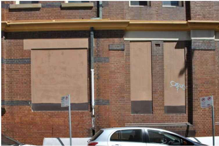
Figure 33. The 1930 addition was designed to sit comfortably with the earlier part of the building, and this has been so successfully achieved that the two parts are only readily discerned on close inspection. Indicators include the clearly defined joint (no attempt was made to key the brickwork) and the subtle differences in the modelling and fenestration of the two sections.
