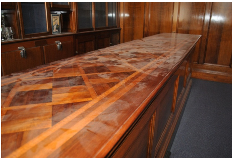
Figure 47. Parquetry bar in the Show Bar – early photographs reveal that the floor was also parquetry laid in the same pattern. It is not known if it survives under the carpet.
