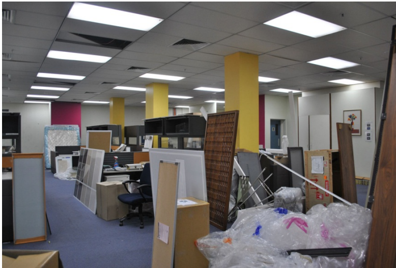
Figure 43. The ground floor has been converted into an open plan office space. Little evidence of the original fabric can be seen.
