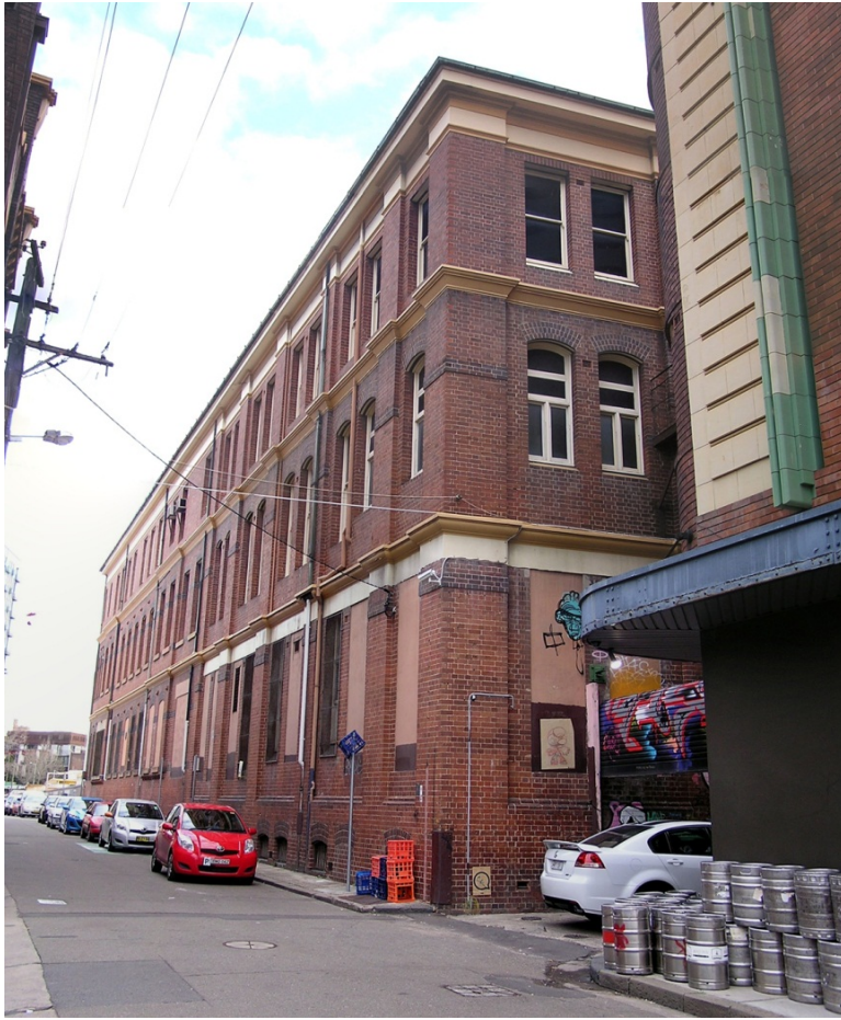
Figure 21. Looking south from Broadway along Kensington Street to the Administration Building.
