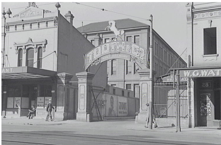
Figure 17. View of the restaurant showing its relationship to the main gateway entrance to the brewery and the brewery's Administration Building to the rear. The shops and gates were demolished in 1939 to facilitate the widening of George Street (Parramatta Road). (Sydney City Council Demolition Photographs (dated 1930s). Sydney City Council Archives Reference Collection 3323.)
