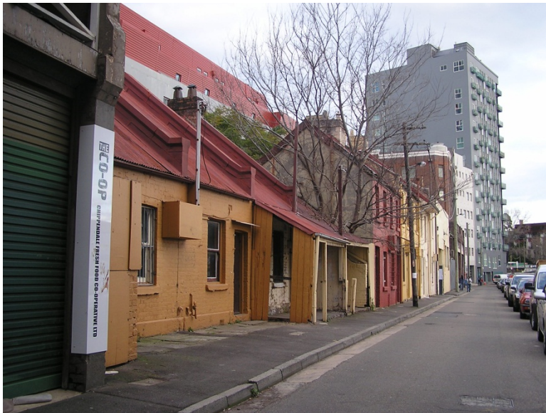
Figure 22. The Administration Building forms part of the historic Kensington Street Precinct.
