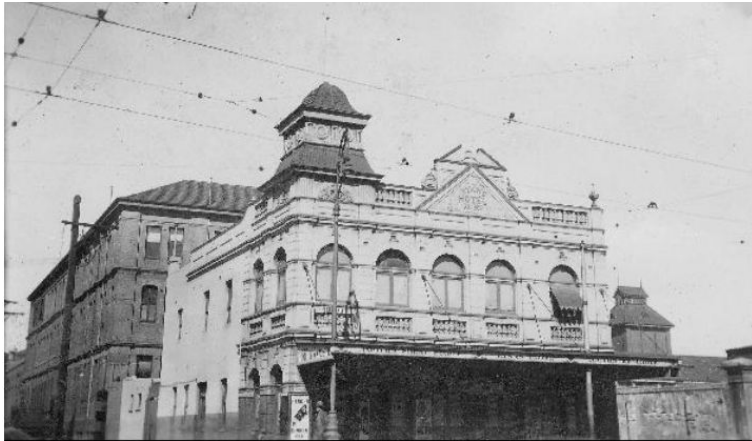
Figure 14. Ryan's Hotel prior to demolition. The form of the extended Administration Building can be seen behind. The adjacent restaurant building at 24 Parramatta Road has been demolished. (Australian National University, Archives of Business and Labour. Tooth & Company Collection. Ref. N60-YC-6. Image date Aug 1939. http://hdl.handle.net/1885/48787 )
