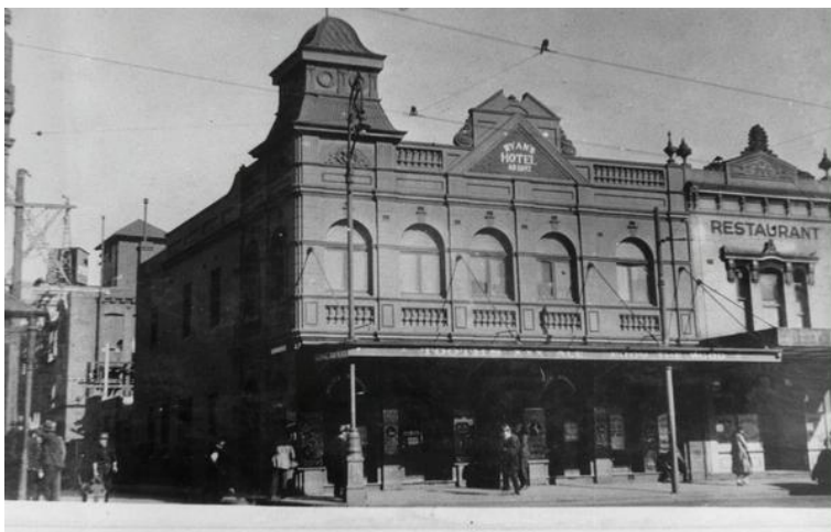
Figure 13. Ryan's Hotel. Building works associated with the major extension to the Administration Building can be seen in the background. (Australian National University. Archives of Business and Labour. Tooth & Company Collection. Ref. N60-YC-6. Image date Aug 1939. http://hdl.handle.net/1885/46193 )
