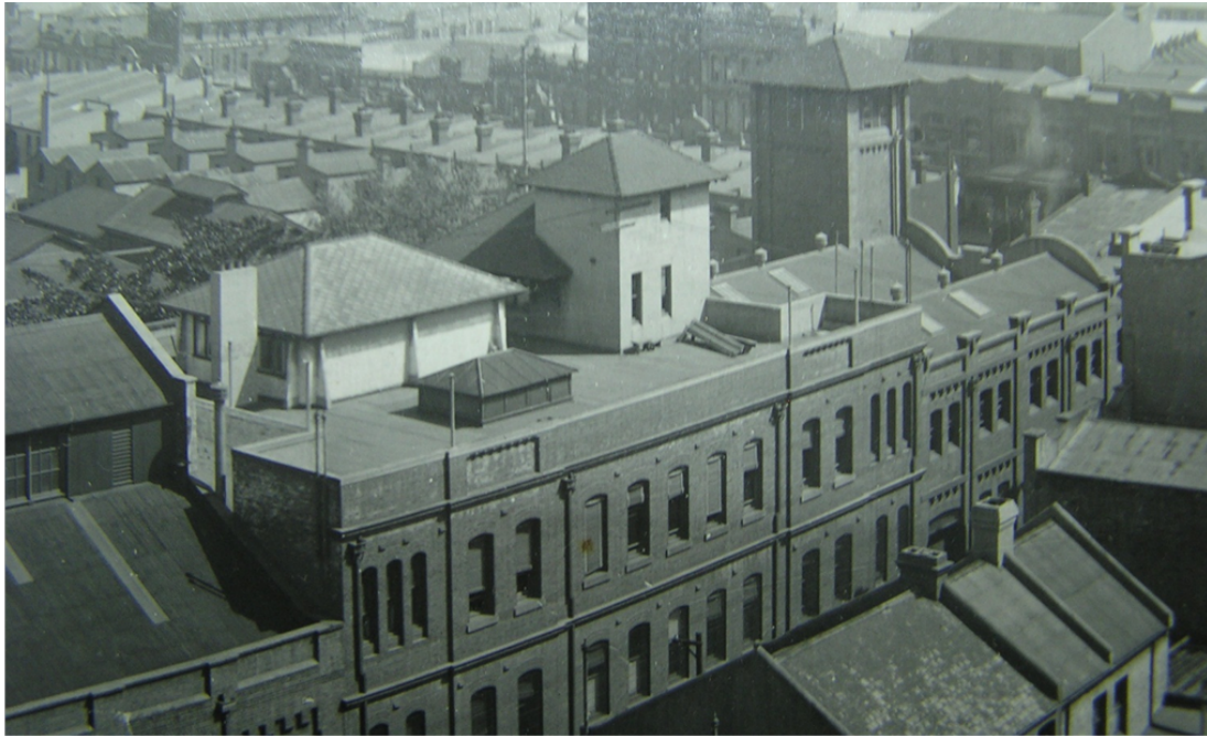
Figure 9. Aerial photograph taken c.1925 showing the original form of the Administration Building with the separate Aerated Waters Factory to the north. Note the two-storey form and flat roof to the Administration Building and the tower to the Aerated Waters Factory. The Aerated Waters Factory was built in the Federation Free Style with a prominent curved parapet facing the Parramatta Road elevation, although the elevation to Kensington Street was more consistent with the traditional 'house' style for brewery buildings. The Aerated Waters Factory building included a cart dock that provided direct access to Kensington Street from the factory – the entrance can be seen at ground level between the two chimneys above the terrace houses. (Tooths Collection: Powerhouse Museum)
