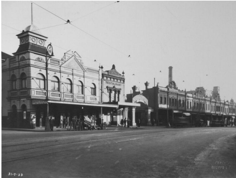
Figure 12. Looking south-west along George Street (Parramatta Road) from Kensington Street prior to the demolition of the buildings to allow the widening of Parramatta Road in 1939. Ryans Hotel is on the left side, and the Restaurant can be seen adjacent to the original entrance gates. (Sydney City Council Demolition Photographs (dated c1933). Sydney City Council Archives Reference Collection. NSCA 51/4572)
