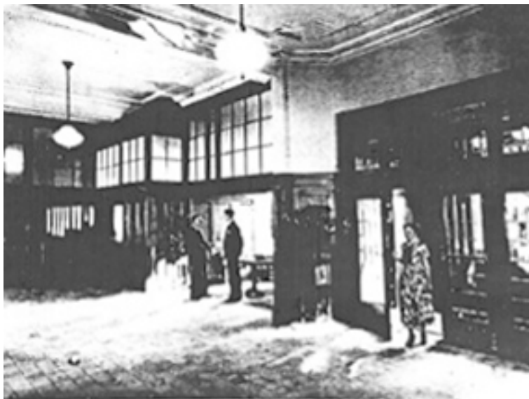
Figure 11. The main vestibule after its remodelling as part of the 1930s works.
