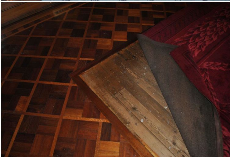
Figure 30. The parquet, although visually rich, is limited to a band around the perimeter of the room, with the centre area (and concealed by the large carpet area) laid in simple unfinished floorboards. The construction of the additional levels to the building will mean that the upper levels will need to be supported during construction, requiring the insertion of supports through the ceiling of the room. These will be made in the parts of the room with raw timber floor, and will align with the plain panels in the ceiling.
