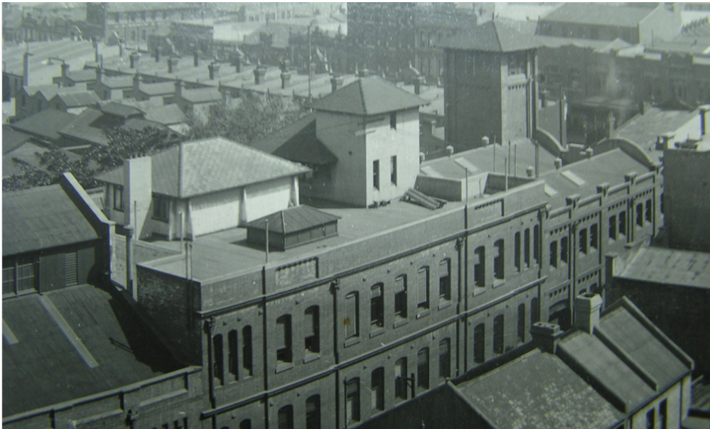
Figure 3. Aerial photograph taken c.1925 showing the original form of the Administration Building with the Aerated Waters Factory to the north. Note the two-storey form and flat roof to the Administration Building and the tower to the Aerated Waters Factory. The Aerated Waters Factory was built in the Federation Free Style with a prominent curved parapet facing the Parramatta Road elevation. The elevation to Kensington Street was more consistent with the traditional 'house' style for brewery buildings. The Factory also included a cart dock that provided direct access to Kensington Street – the entrance can be seen at ground level between the two chimneys above the terrace houses. (Tooths Collection: Powerhouse Museum)
