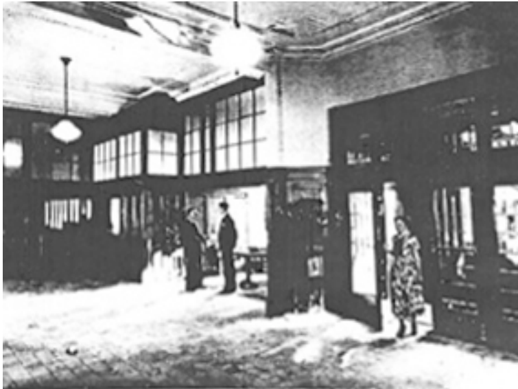
Figure 5. The main vestibule after its remodelling in the 1930s works. Image Museum of Applied Arts and Science (Powerhouse Museum) PH 28 86/3769. (Sourced from 1991 CMP by Planning Workshop and Associates)
