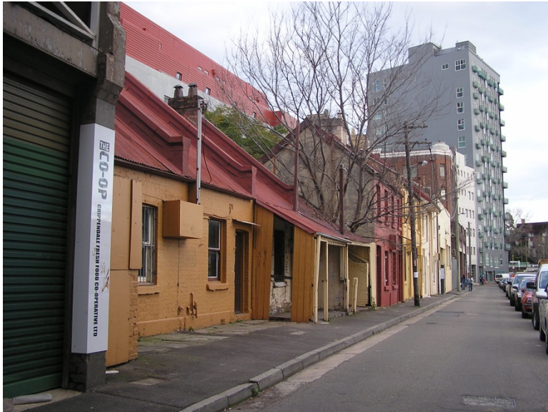
Figure 10 The Administration Building forms part of the historic Kensington Street Precinct.
