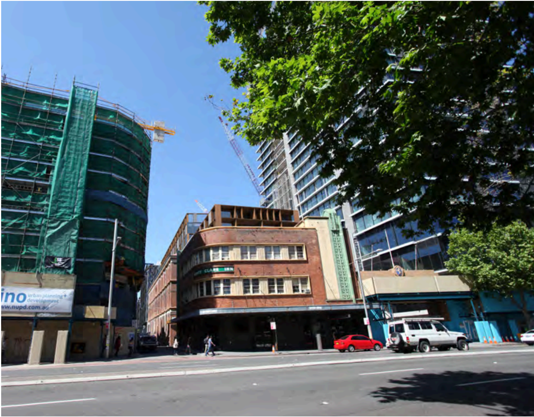
1 - VIEW OF NORTH ELEVATION FROM BROADWAY
