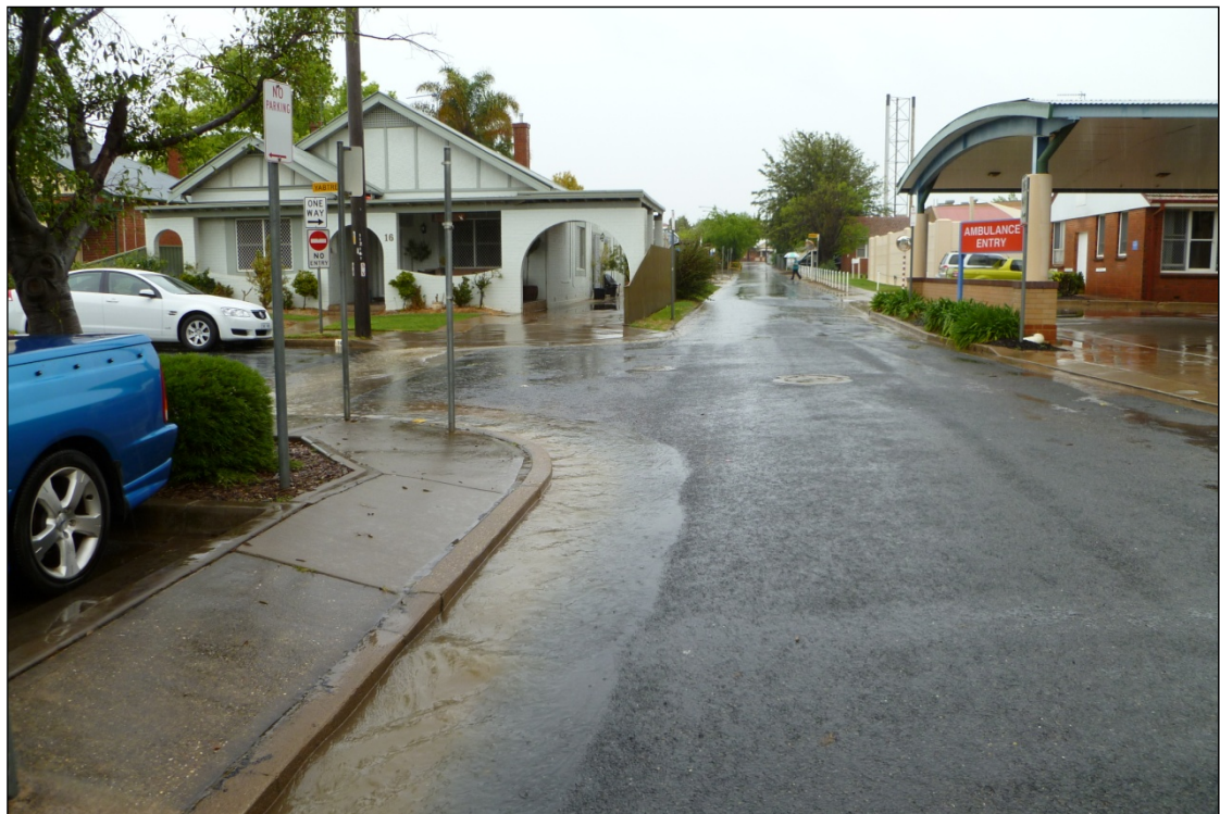
Figure 2.2 – Lewis Drive Gutter Flow
